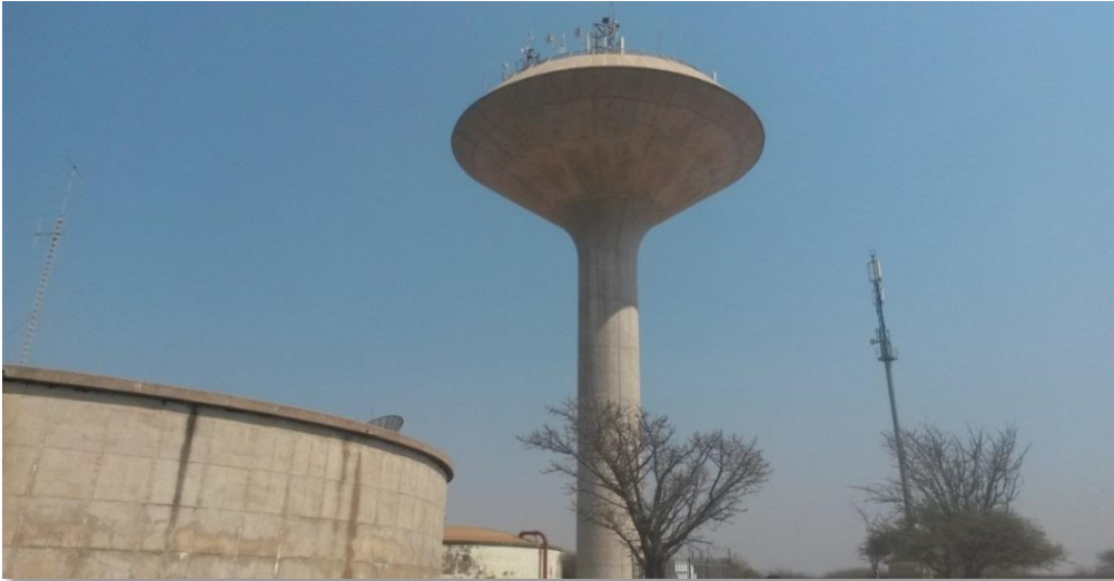
Figure 12- Bosveldsig ground level reservoir and water tower
