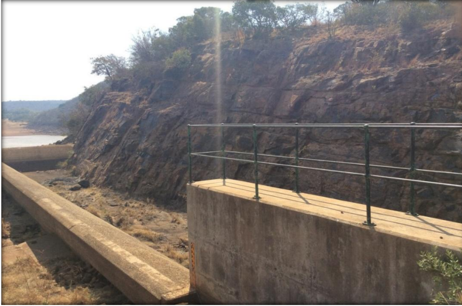
Figure 8 -Donkerpoort Dam overflow weir flanked by the cliff
