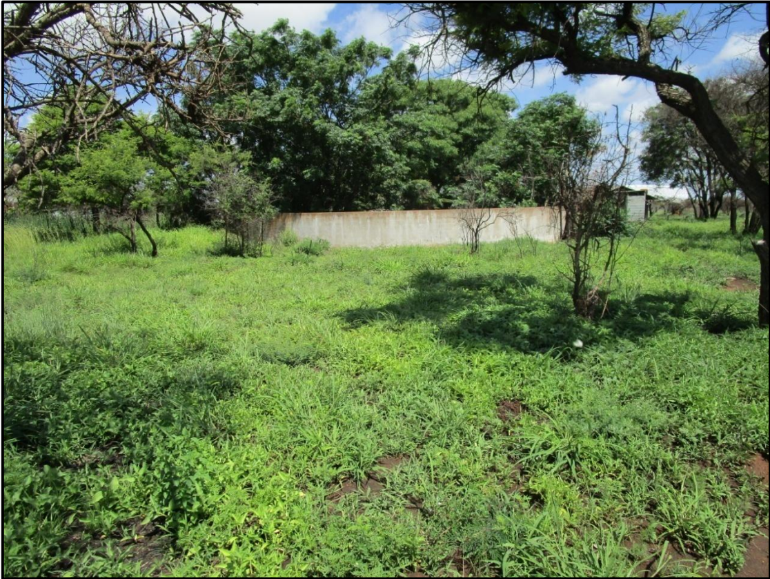
Figure 9. View of a reservoir – the opposite side has collapsed.
