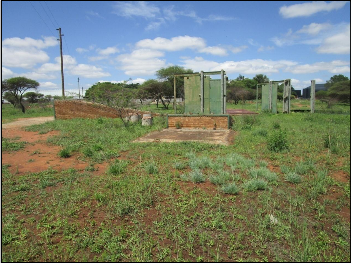
Figure 8. View of the loading structures at the stock pen.
