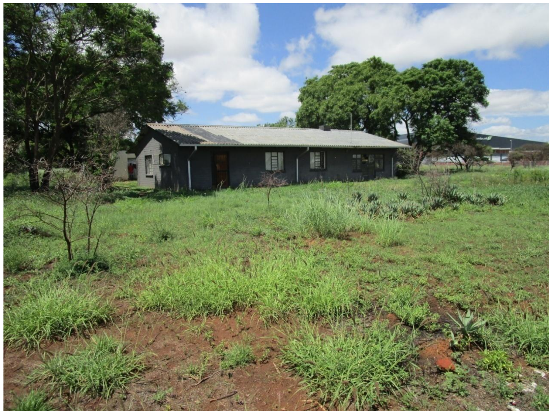
Figure 5. View of the residential dwelling on the property.
