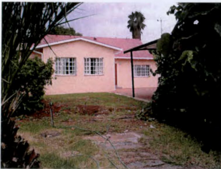
Photo 2: View of altered North façade.
