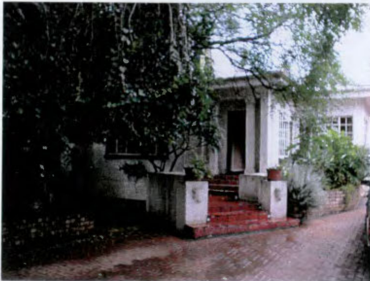
Photo 2: House viewed from North West showing the entrance.
