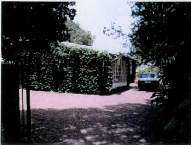
Photo 2: View from the North East.
