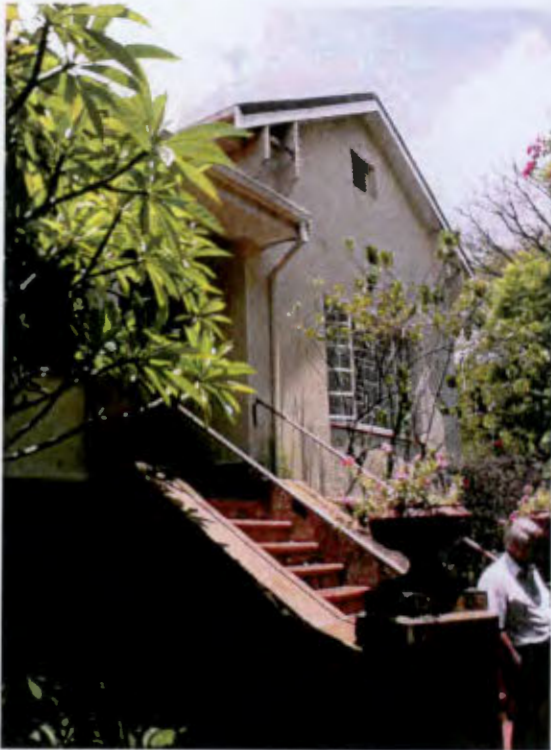
Photo 3: North façade and entrance of the house
