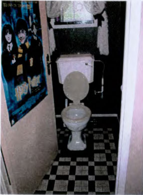
Photo 1: Original bathroom fittings and tiling.
