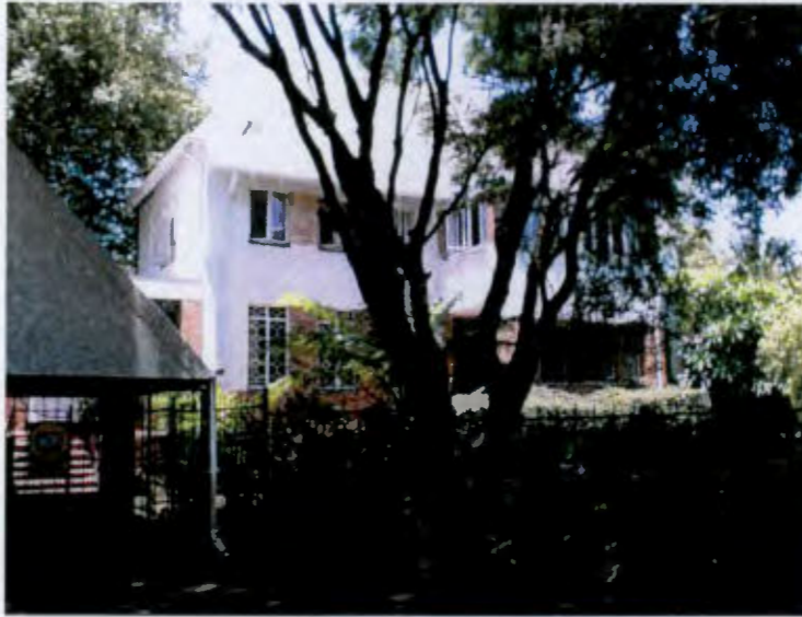
Photo 1: View of house from the North.
