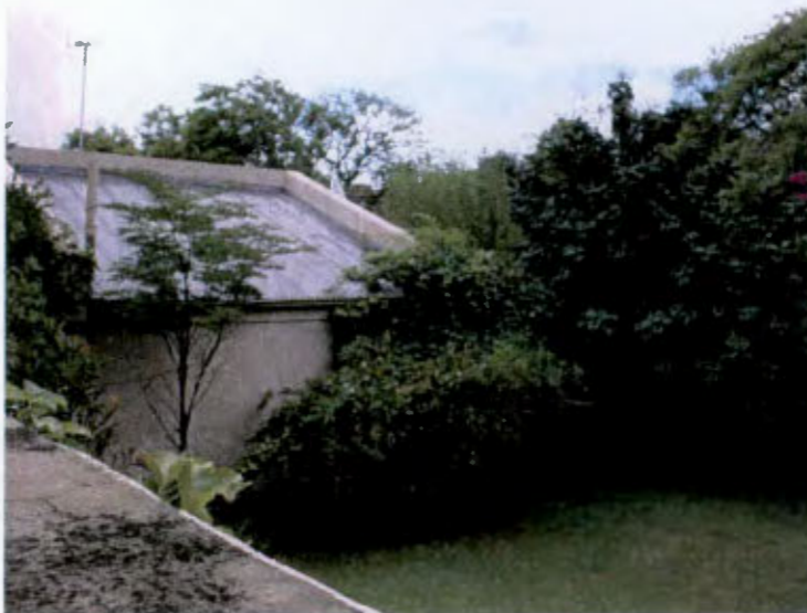
Photo 2: View over panhandle boundary wall.
