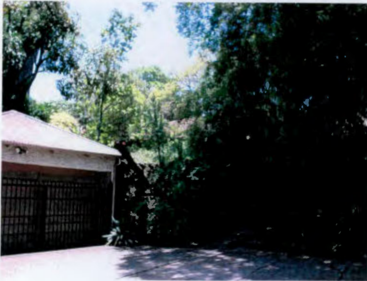
Photo 2: Original garage adjacent entrance off Loveday St.
