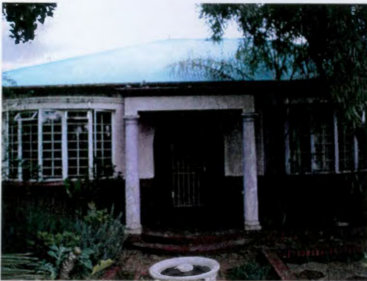
Photo 2: Porch and bow windows on East façade from the East.
