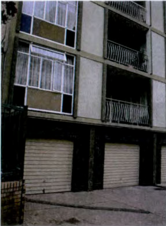
Photo 1: Basement garages on North façade.
