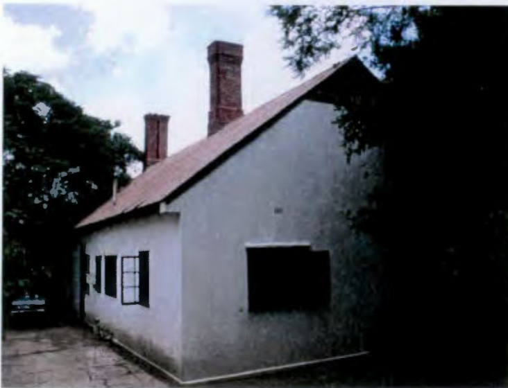
Photo 2: View of the house from the South East.
