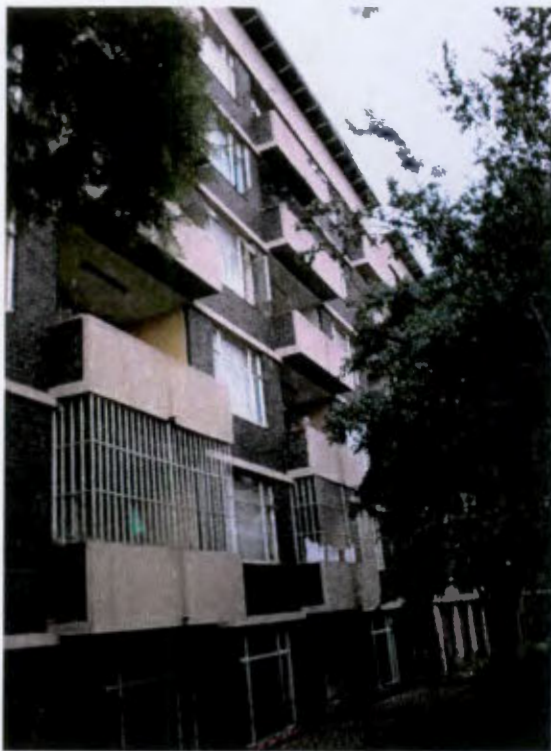
Photo 1: North façade showing infill obscuring ground floor pilotis.
