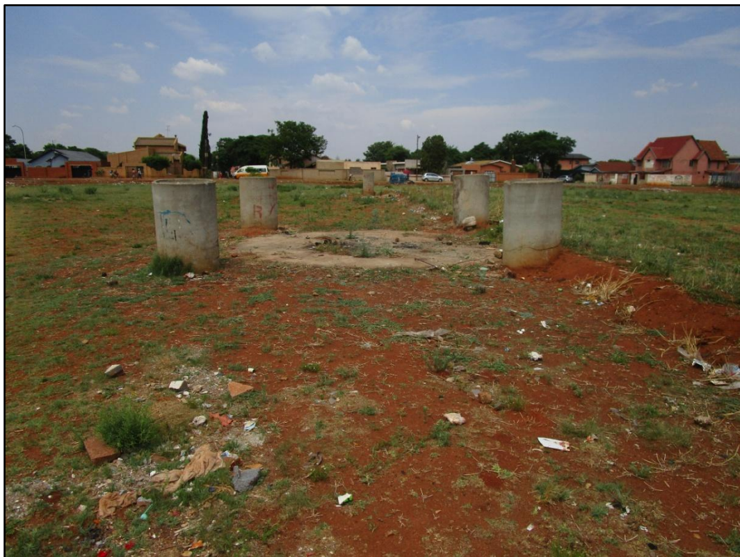
Figure 2. A view of the structure on the terrain made from concrete pipes.
