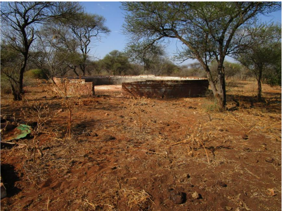
Figure 10. View of large brick and cement reservoir.
