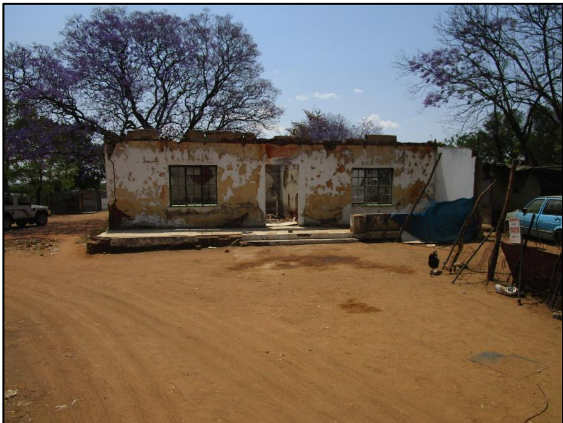
Figure 12. View of partially demolished structure at cluster 4.
