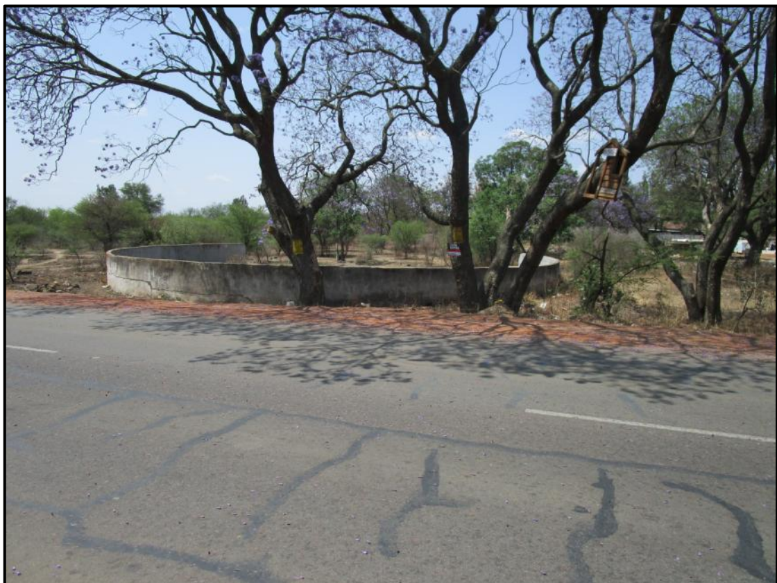
Figure 14. View of old reservoir on Smallholding 78.
