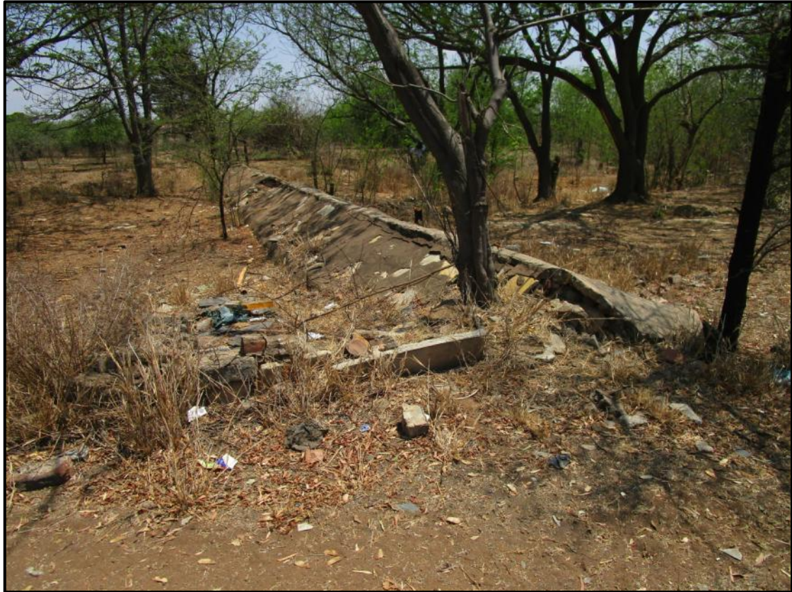
Figure 13. View of a weir in the drainage line.
