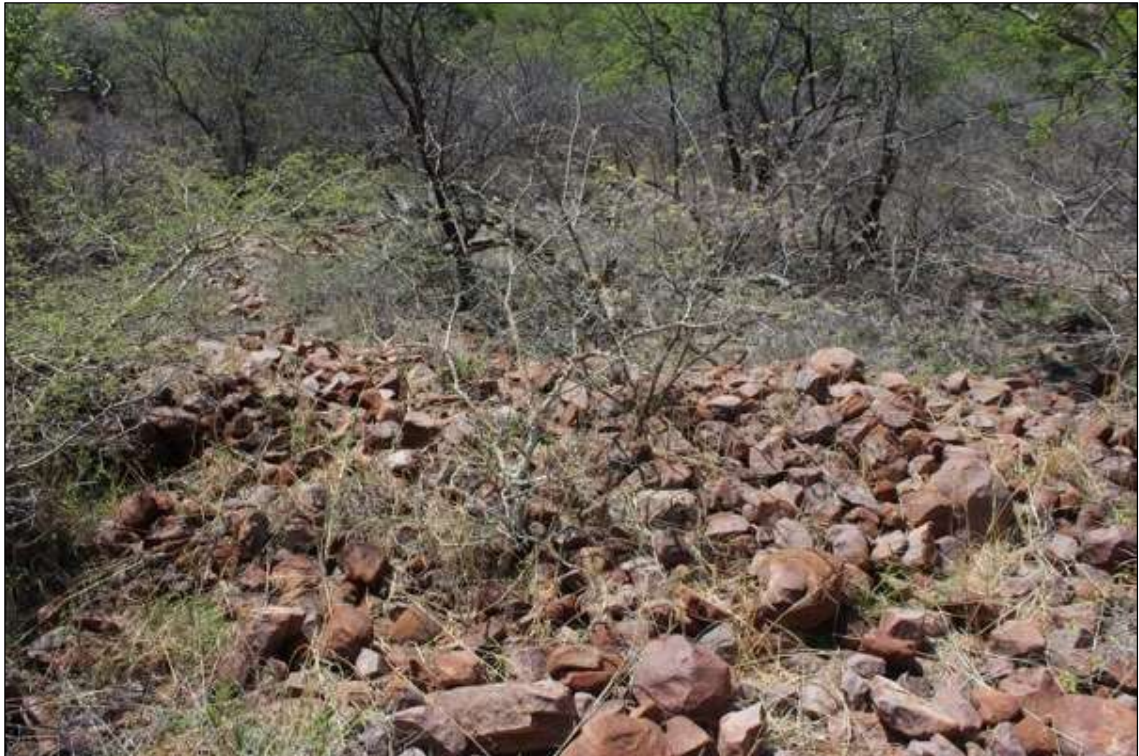
Figure 25: Collapsed stone walls at the bottom slope of the mountain
