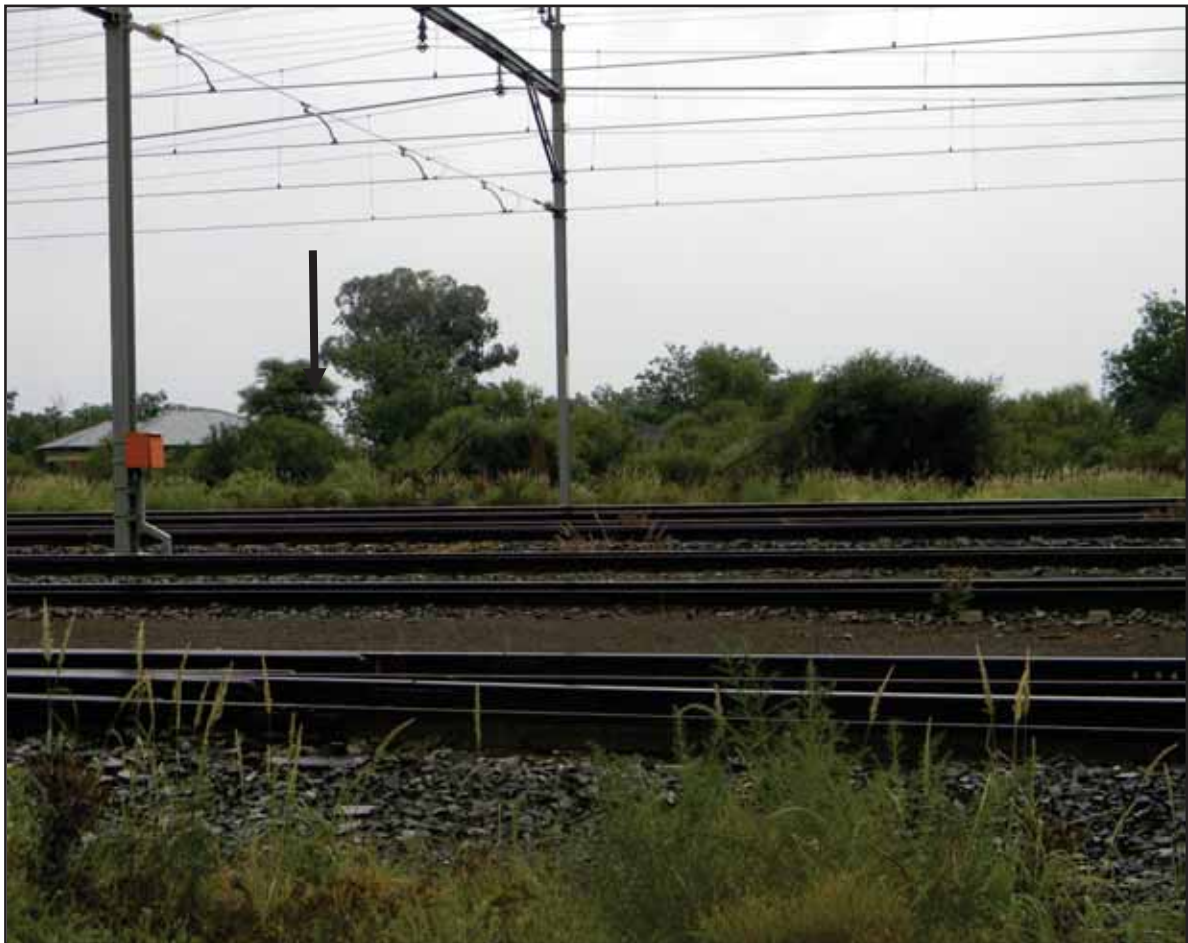
Figure 52: Historical railway structures and railway within the reserve at Ulco Station
