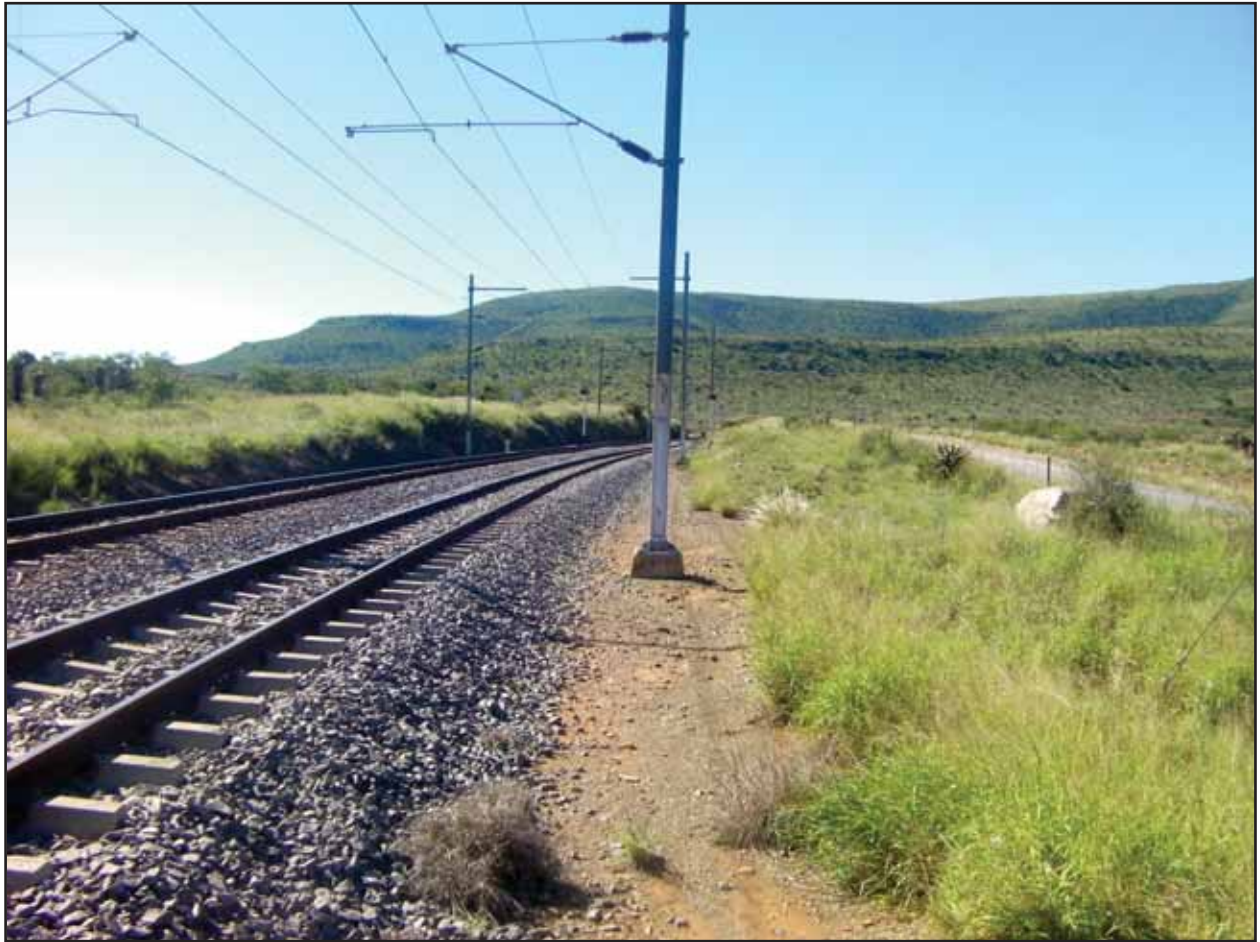
Figure 80: Cookhouse to Drennan
