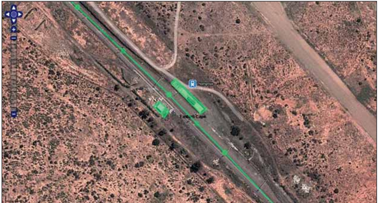
Figure 78: Thorngrove Station evident of old railway buildings (SAHRIS, 2013)
