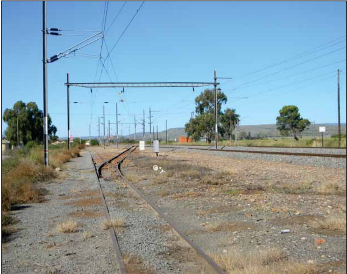
Figure 83: Railway infrastructure at Golden Valley Station
