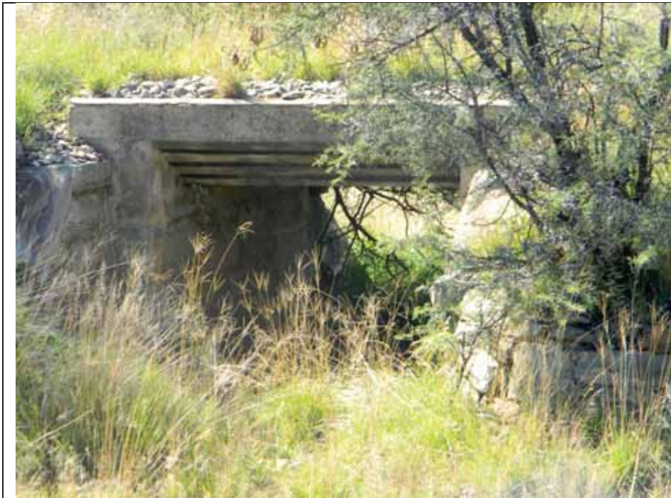
An example of a culvert that occurs in the Eastern Cape section
