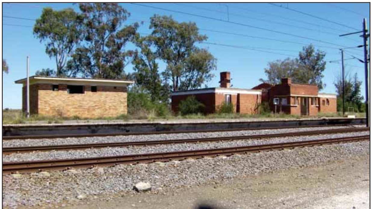
Figure 92: Old railway buildings at Sheldon
