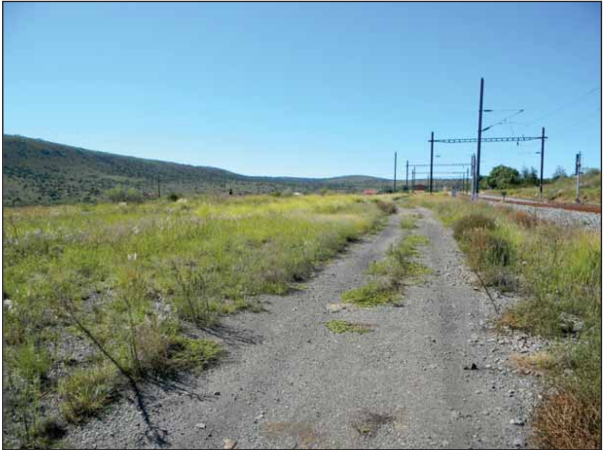
Figure 96: Railway reserve road heading towards Kommadagga Station
