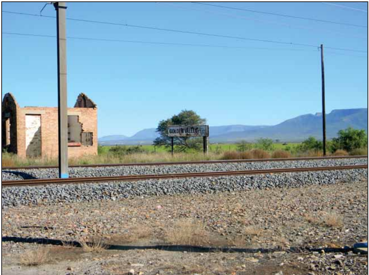
Figure 81: Golden Valley Station and historical structures
