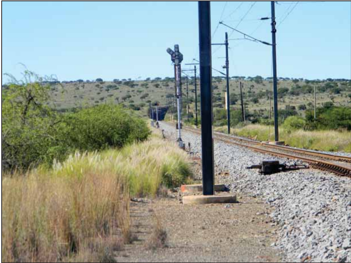
Figure 102: Railway line positioned south of Kommadagga Station
