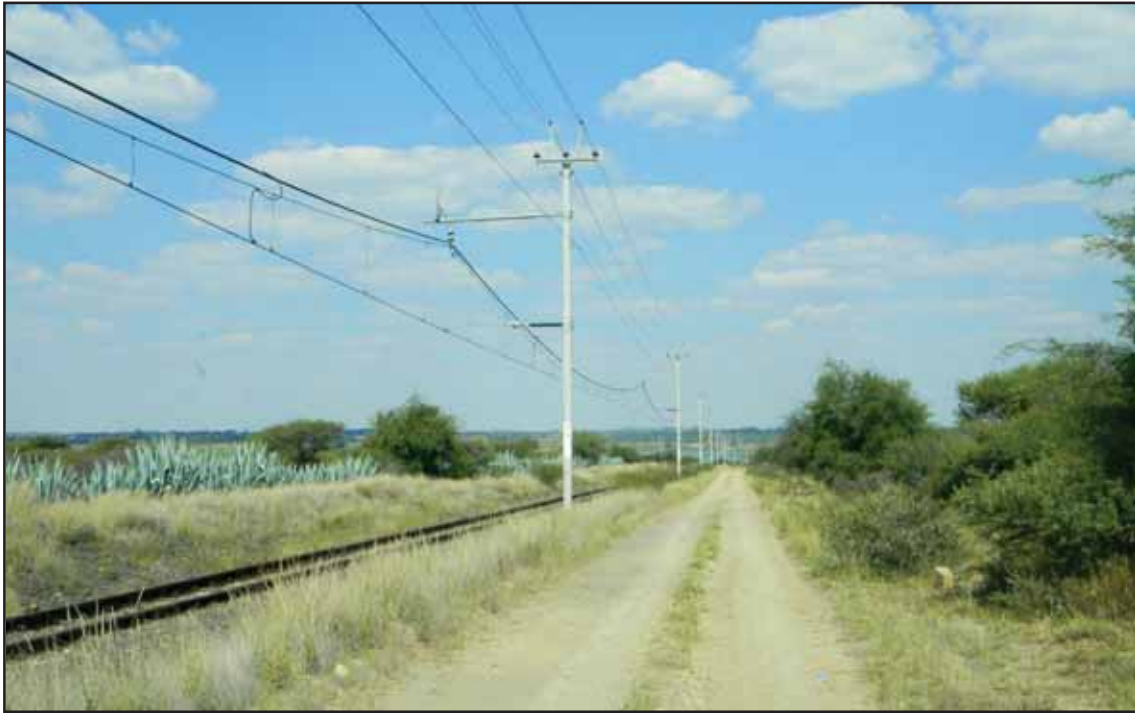
Figure 69: The railway reserve south of Fieldsview Station
