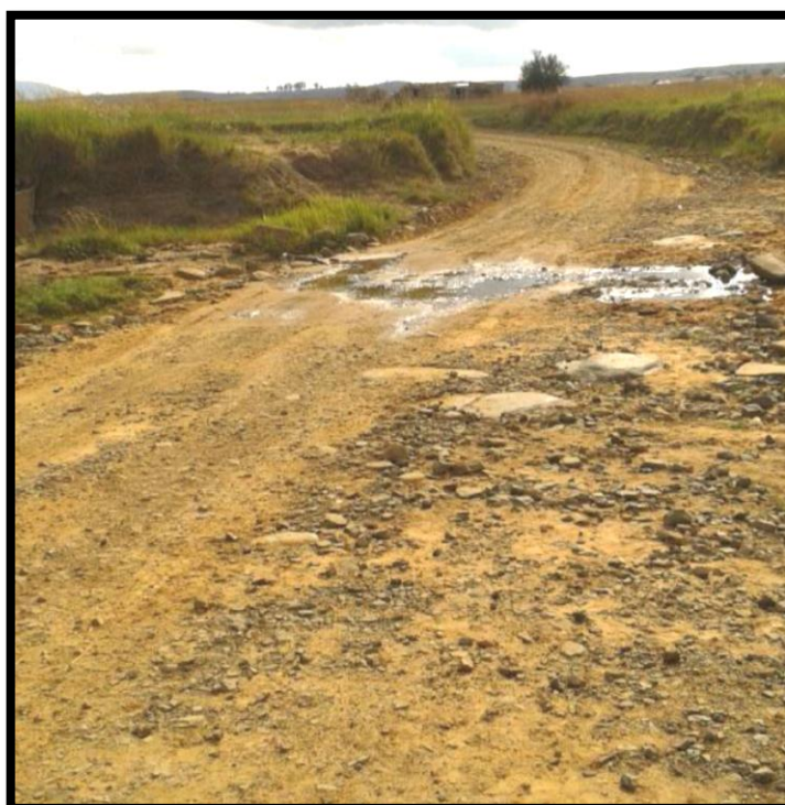
Figure 4. Access Road L2957 showing dongas and alien vegetation adjacent to the road.
