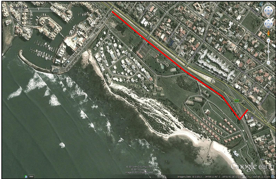
Figure 6: The proposed route along Faure Marine Drive which should be monitored for archaeological heritage.
