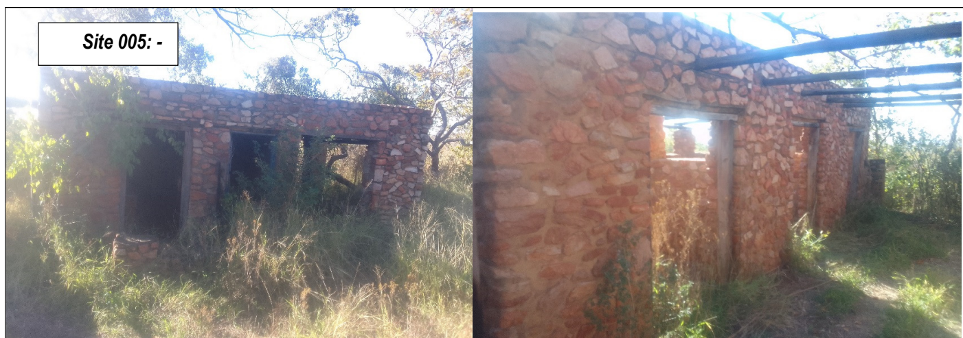
Figure 9: View of a disused servant's quarters
