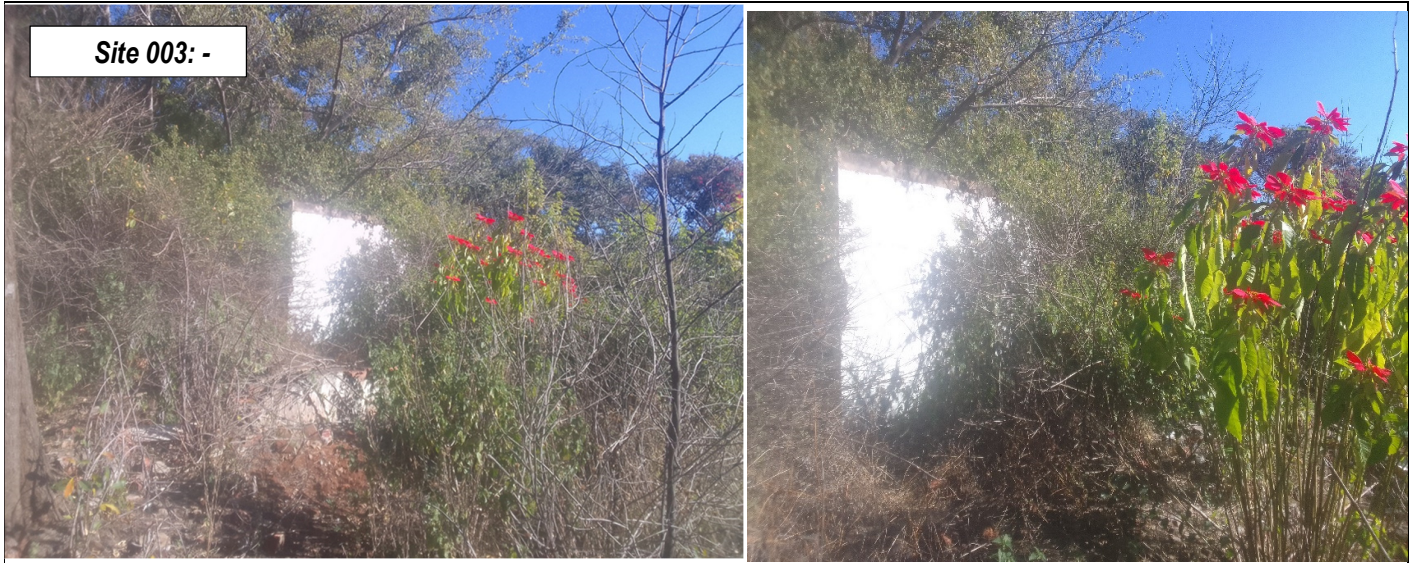
Figure 7: View of the disused water pump station
