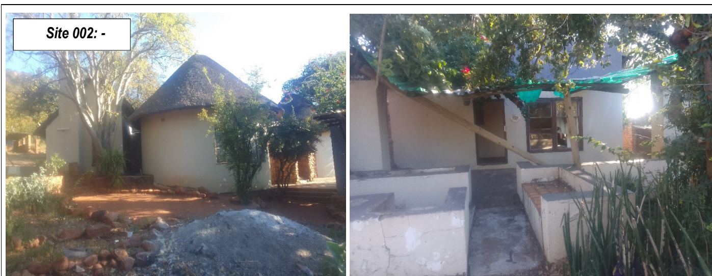
Figure 6:View of the old building / farm house on portion RE/152/445. Note that the farm house has got a few other properties within the same yard. These include a swimming pool and a cartage
