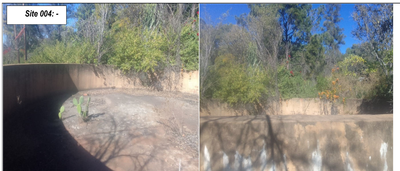
Figure 8: View of a disused water reservoir tank. Note that the tank is still structurally sound
