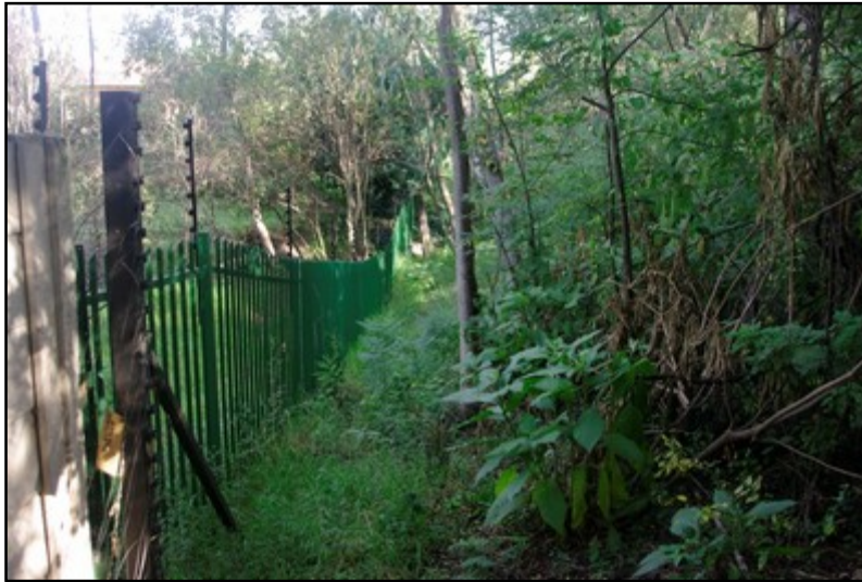
Plate 1: View of the northern extremity of the Sewer Pipeline A study site
