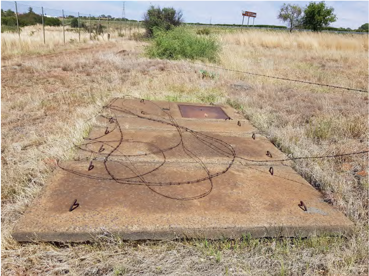
Figure 5: Cements slabs with a metal trapdoor S29° 04' 57.7" E26° 10' 38.5"
