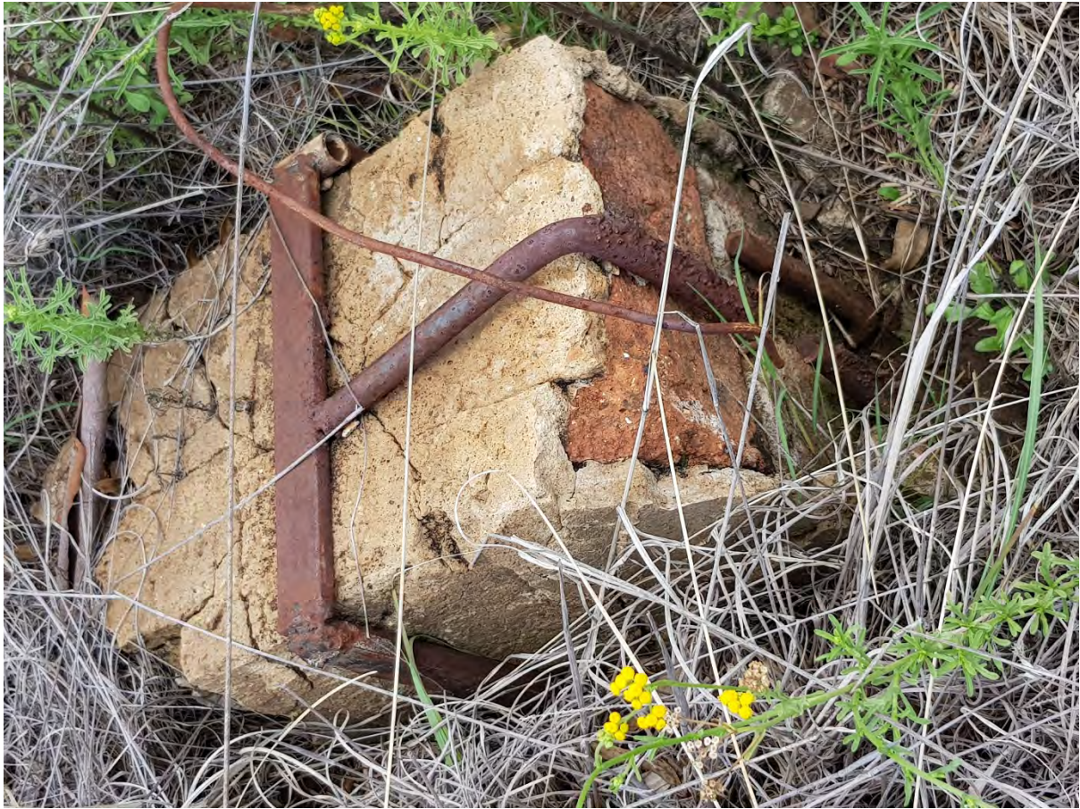
Figure 14: Close-up view of metal brackets
