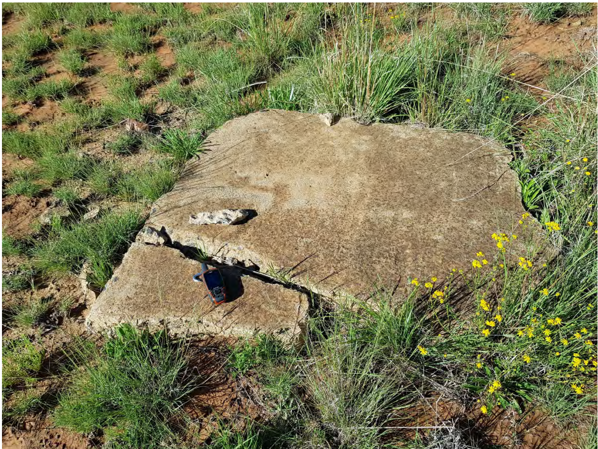
Figure 34: Broken slab of concrete - S29° 05' 13.4" E26° 10' 36.9"
