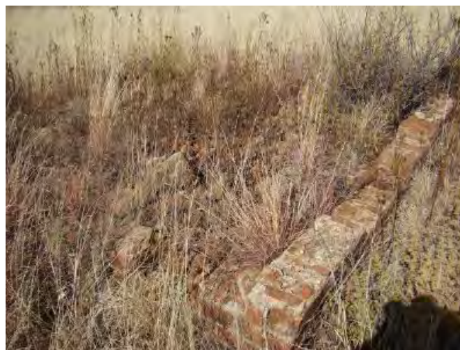
Figure 3: Foundation of historic brick ruin - 2.5 x 3 m
