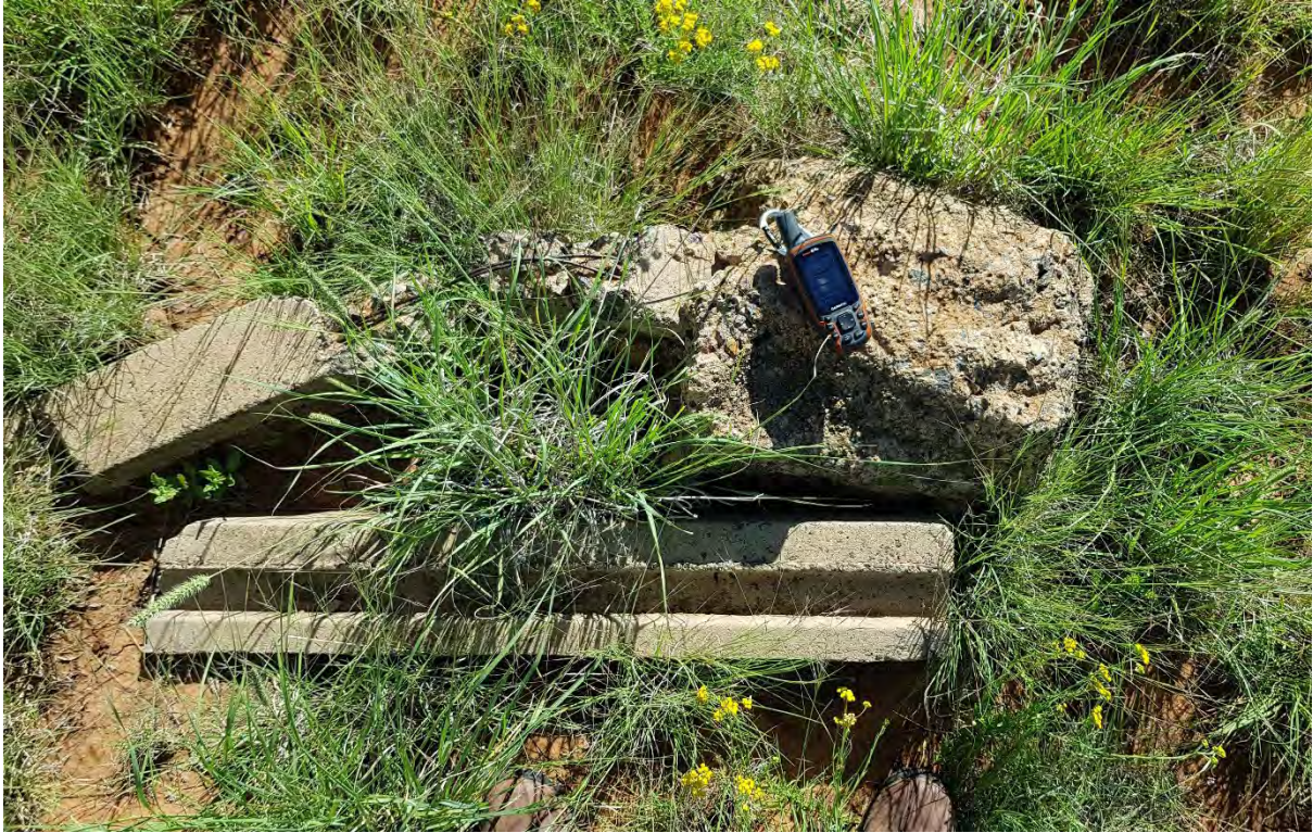
Figure 37: Concrete slabs - top one with two thin metal rods inside -S29° 05' 13.5" E26° 10' 37.6"
