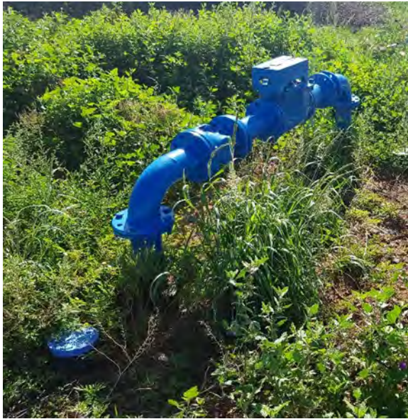
Figure 8: Water pipe S29° 04' 35.4" E26° 11' 28.6"
