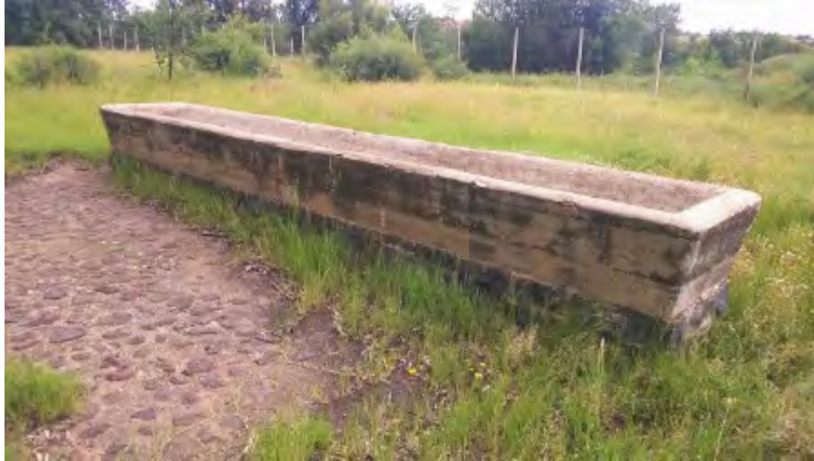
Figure 2: Brick troughs - 100 cm (width) X 685 cm (length) x 65 cm (height)
