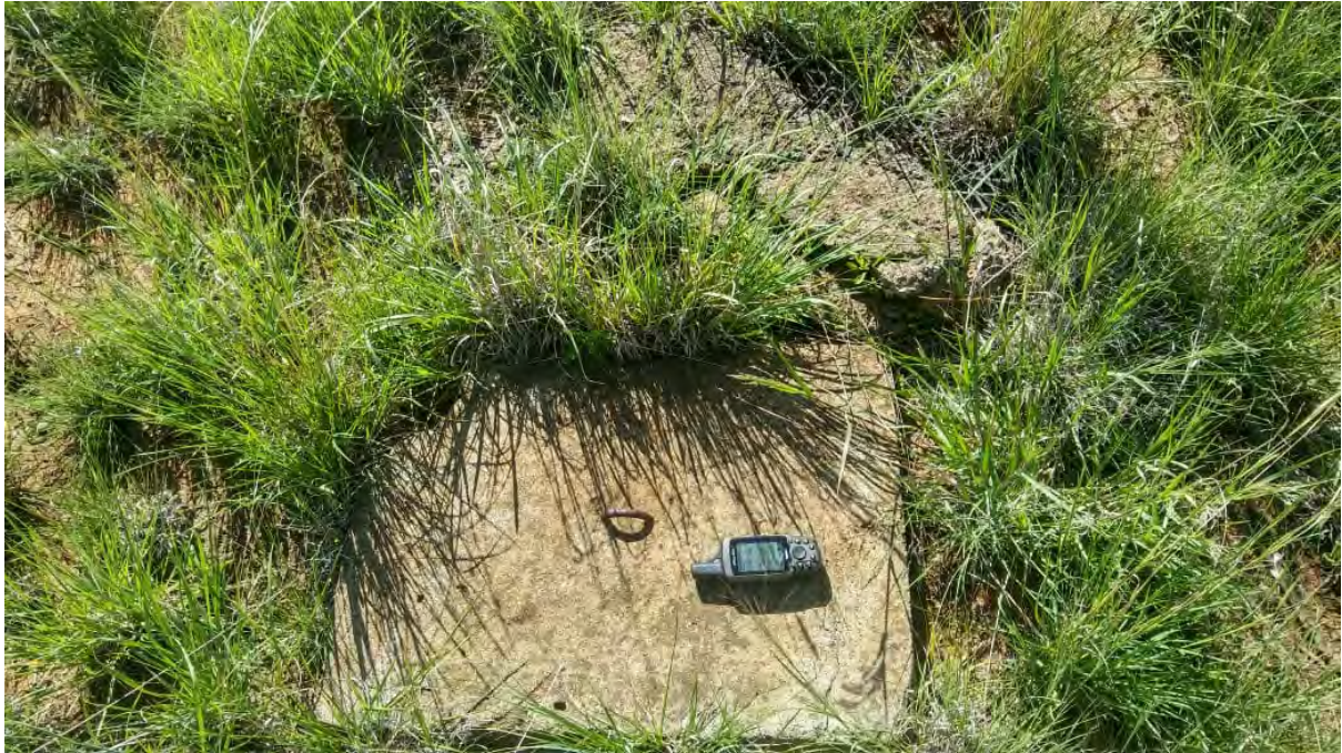
Figure 48: Concrete rubble - including concrete trapdoor -S29° 05' 10.2" E26° 10' 38.8"
