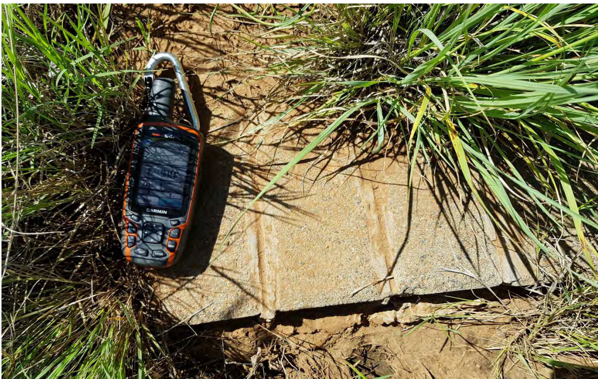
Figure 26: Four cement bricks still attached to each other with mortar. No sign of any foundations in the vicinity. S29° 05' 19.4\"/>
