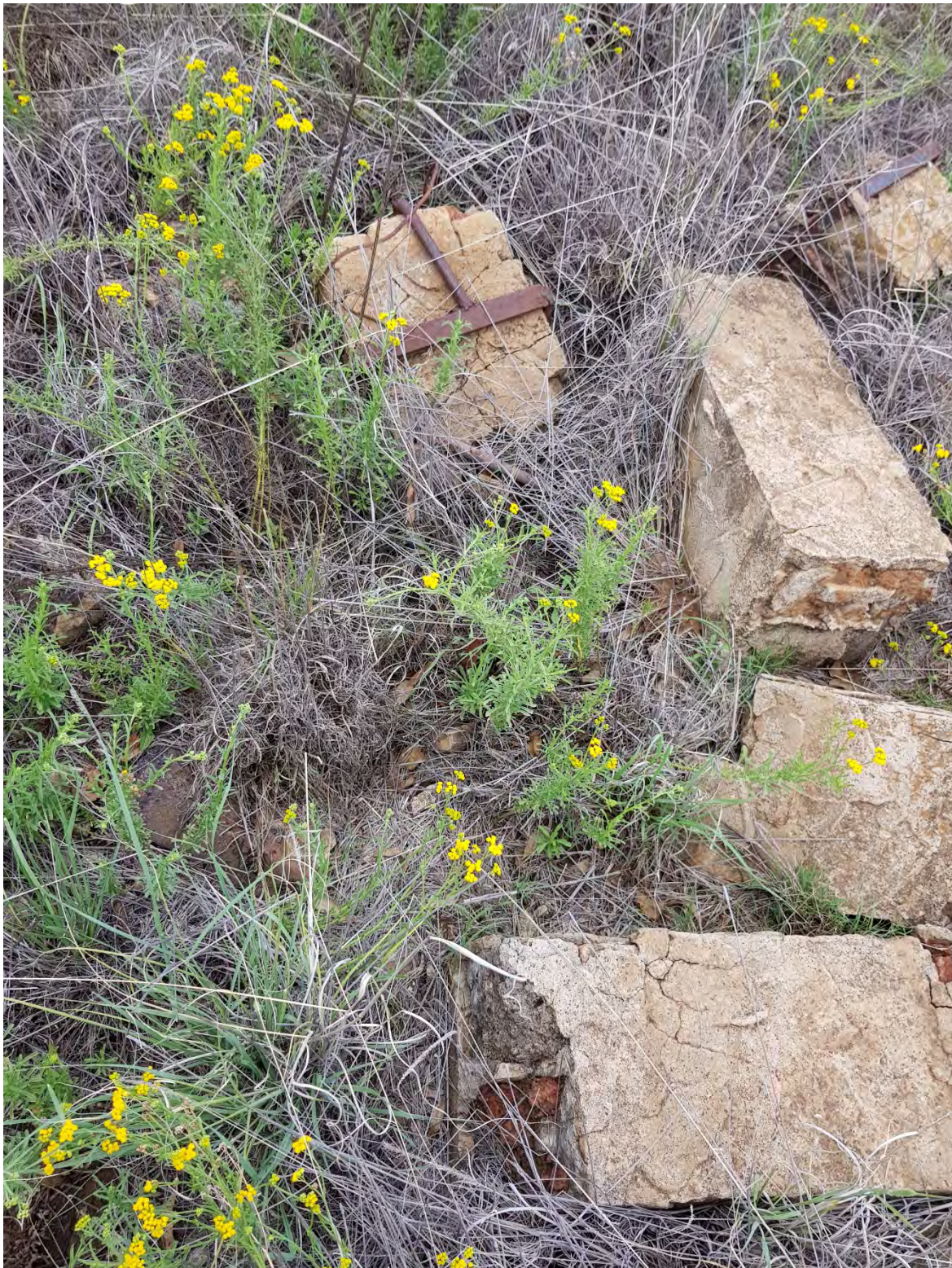
Figure 12: Building rubble, presumably linked with the earlier tempe wall - possibly the pillars of a gate entrance as it is thicker than the wall sections and contains metal brackets that might have served to fix the gate to the pillars - S29° 04' 52.4" E26° 10' 50.8"
