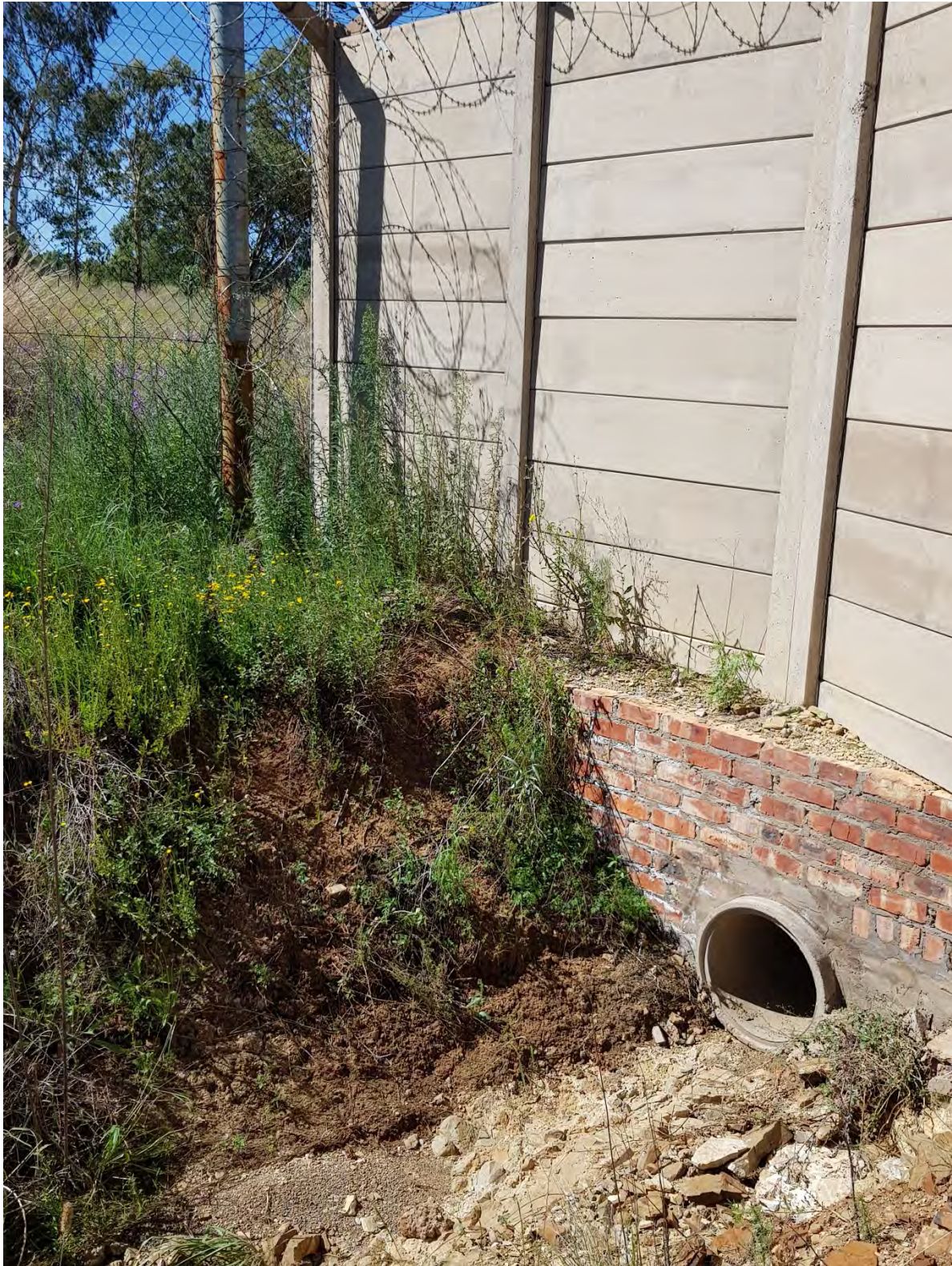
Figure 45: Drain culvert - western corner of Tempe military base -S29° 04' 55.7" E26° 10' 46.1"
