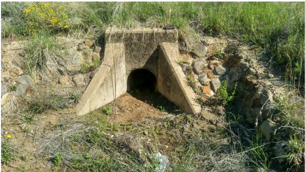
Figure 9: Road drainage culverts (S29° 04' 41.5" E26° 11' 16.1"; S29° 04' 41.0" E26° 11' 15.8"; S29° 04' 42.1" E26° 11' 13.9")
