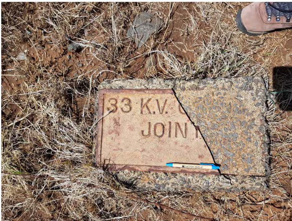
Figure 6: Metal plate fixed on concrete slab - found close to above cement slab structure S29° 04' 57.8" E26° 10' 38.4"
