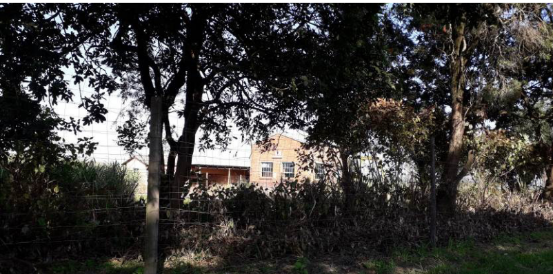
Figure 12 - Treatment plant seen from farmstead 1
