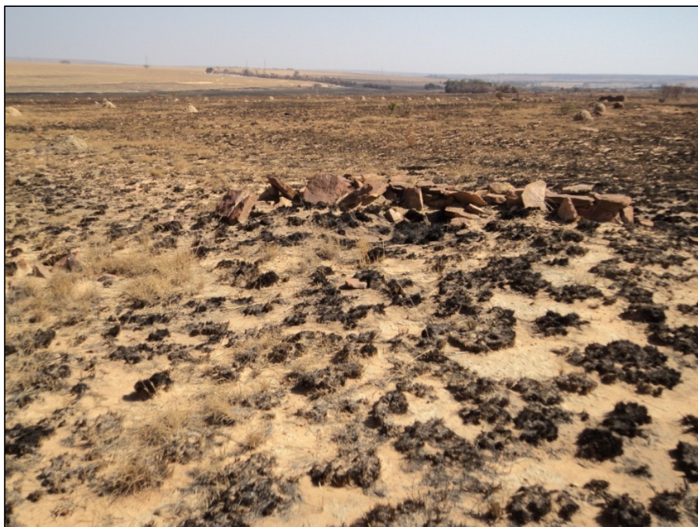
Figure 9: Heritage site PSI-3 (Dilapidated stone wall)
