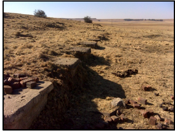
Figure 17: Unknown brick and concrete structure (Site U8)
