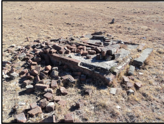
Figure 14: Dilapidated brick Structure (Site U5)
