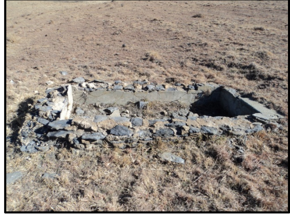
Figure 15: Angular concrete structure (Site U6)
