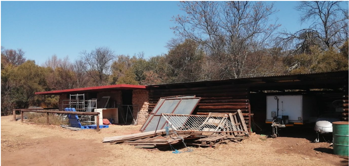
Figure 11: The stables/barn, constructed of stones and tarred poles. Currently used as storage facility.
