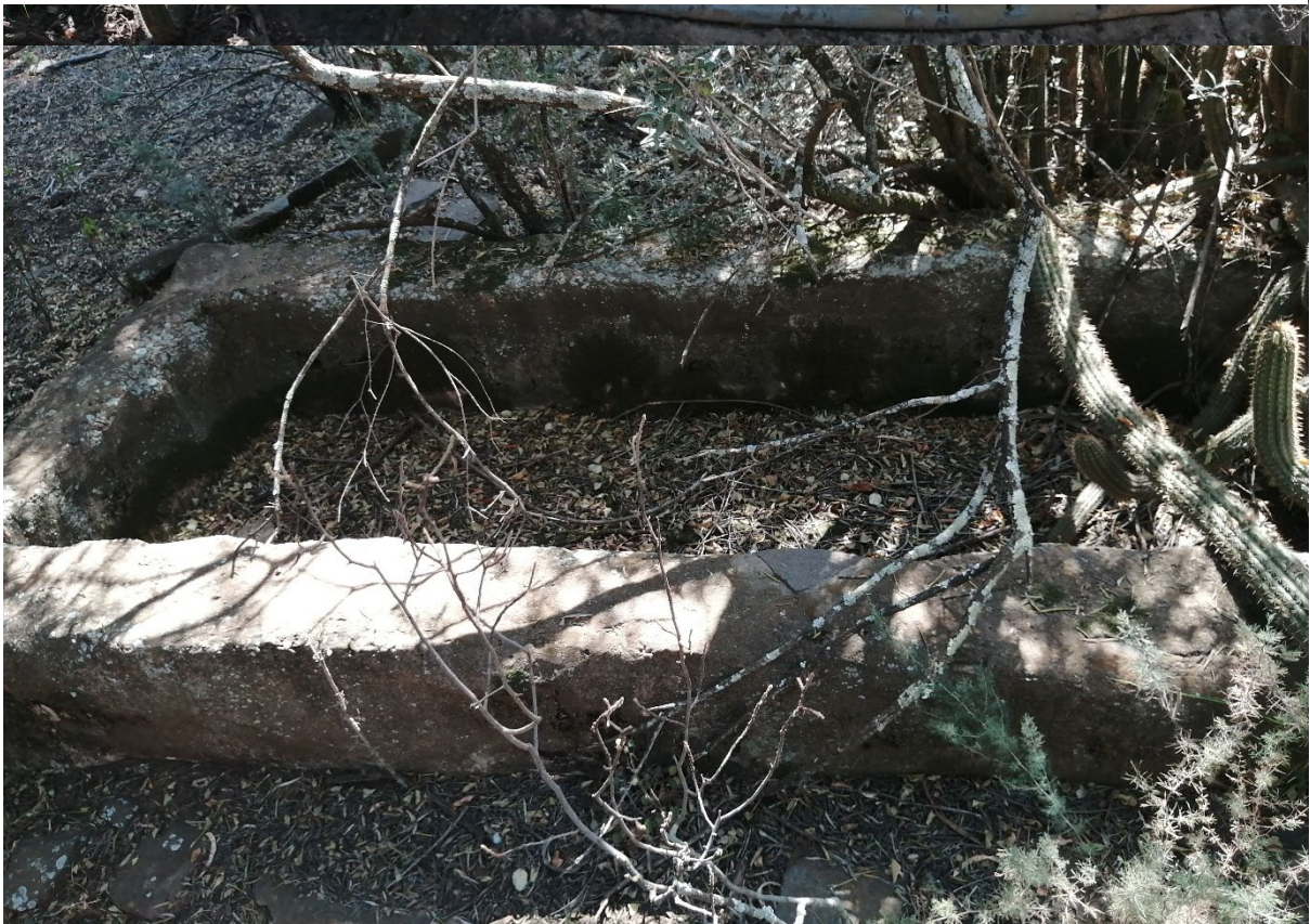
Figure 17: Small trough constructed of stones and cement
