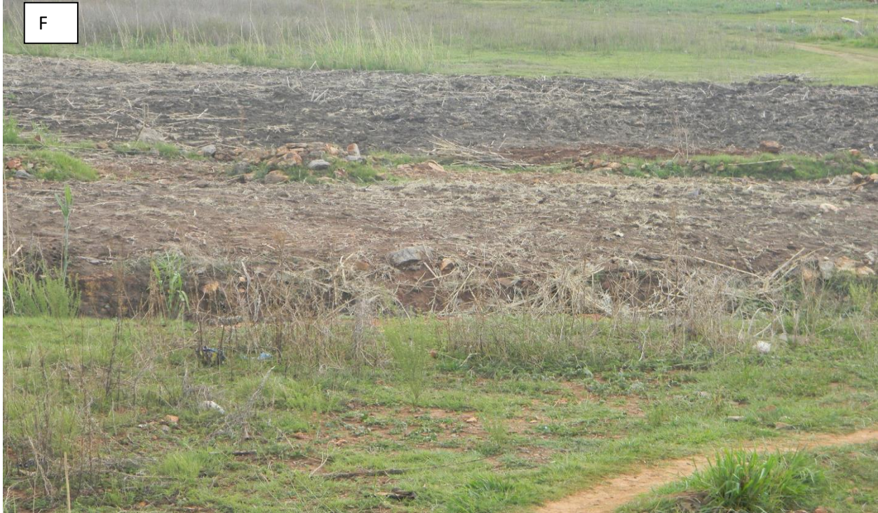
Plate 6: Photo F showing bulk sewer pipeline route (Author 2018).
