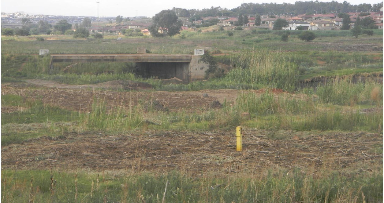
Plate 4: Photo D. showing pipeline bulk sewer pipeline route.
