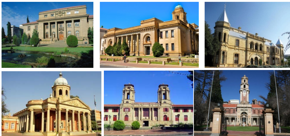
Figure 7: Examples of buildings in Pres Brand Street Conservancy (Clockwise from the top left is the Supreme Court of Appeal, the Free State High Court, the Old Presidency, The National Afrikaans Literary Museum and Research Centre, the City Hall and the Fourth Raadsaal)
