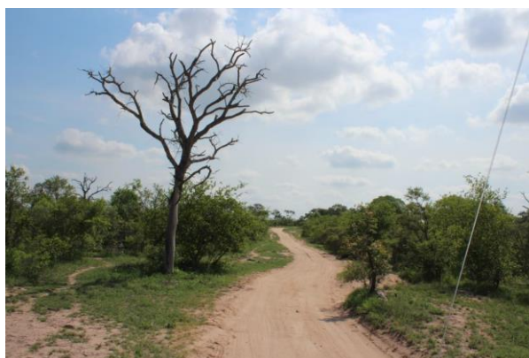
FIGURE 16 A SECTION OF MAIN ROAD WEST THAT IS TYPICAL OF BOTH THAT REQUIRES UPGRADING (© KL Zunckel)
