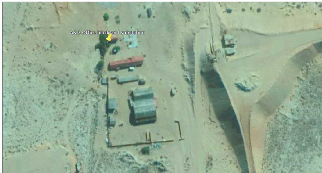
Figure 50. AK3 Office Block and Sub Station
