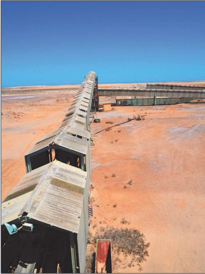
Figure 31. Conveyor Belt System
