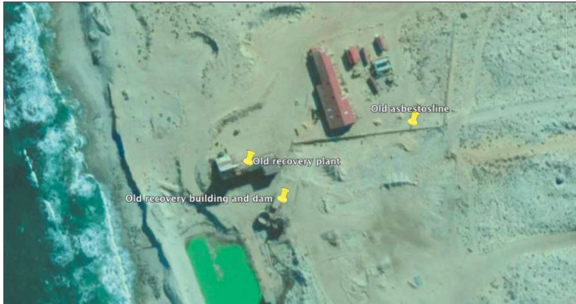
Figure 44. Old Recovery Plant and Asbestos Line
