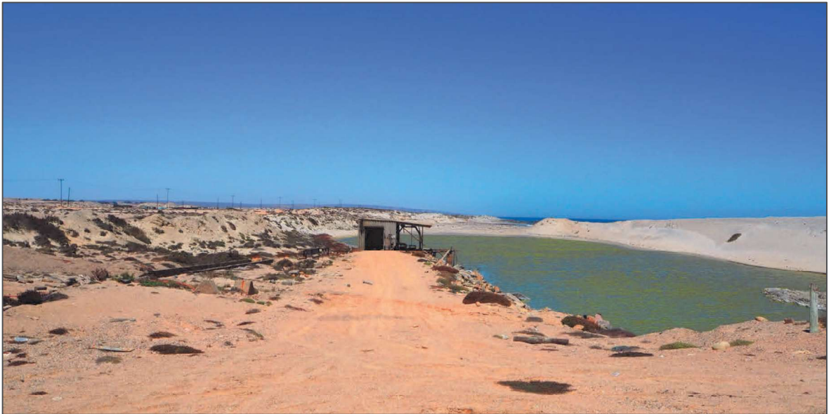
Figure 46. Recovery Plant Dam and Pump Station
