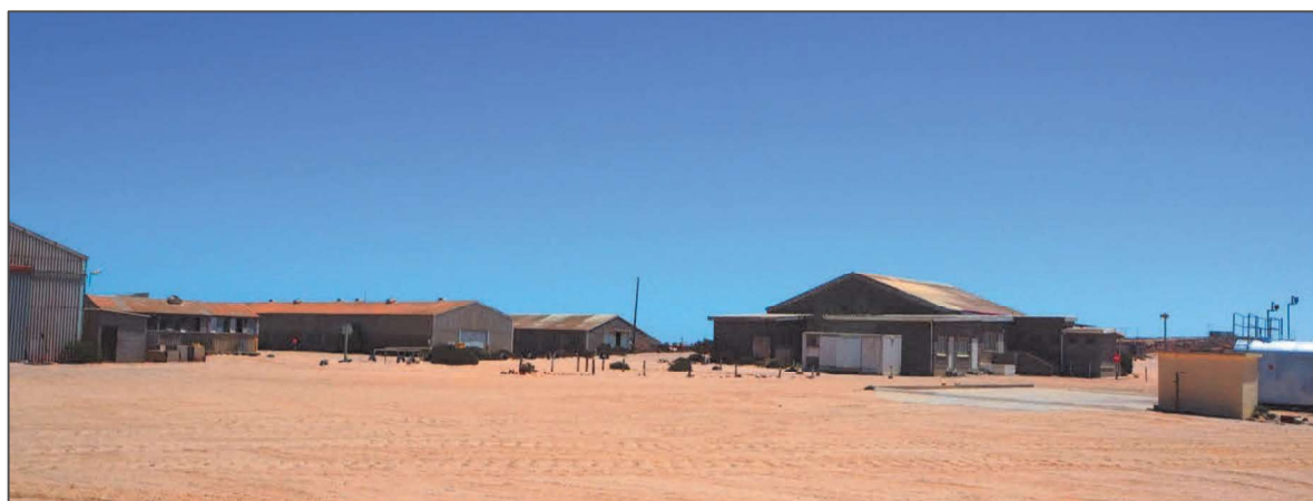
Figure 35. Offices and Workshops
