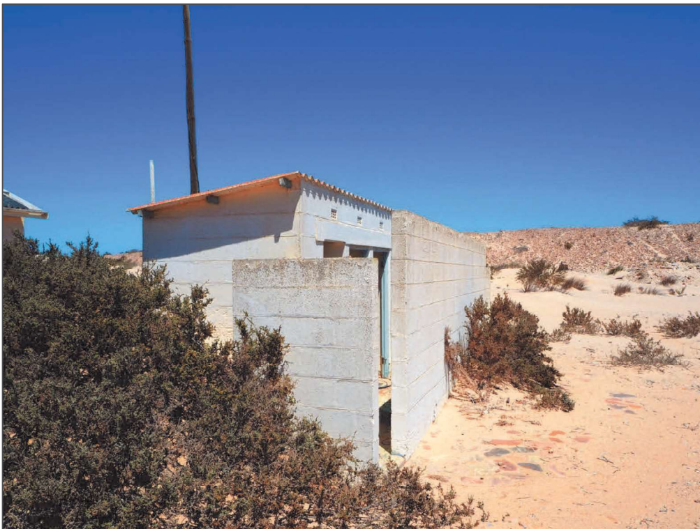
Figure 25. Ablution block Dreyerspan
