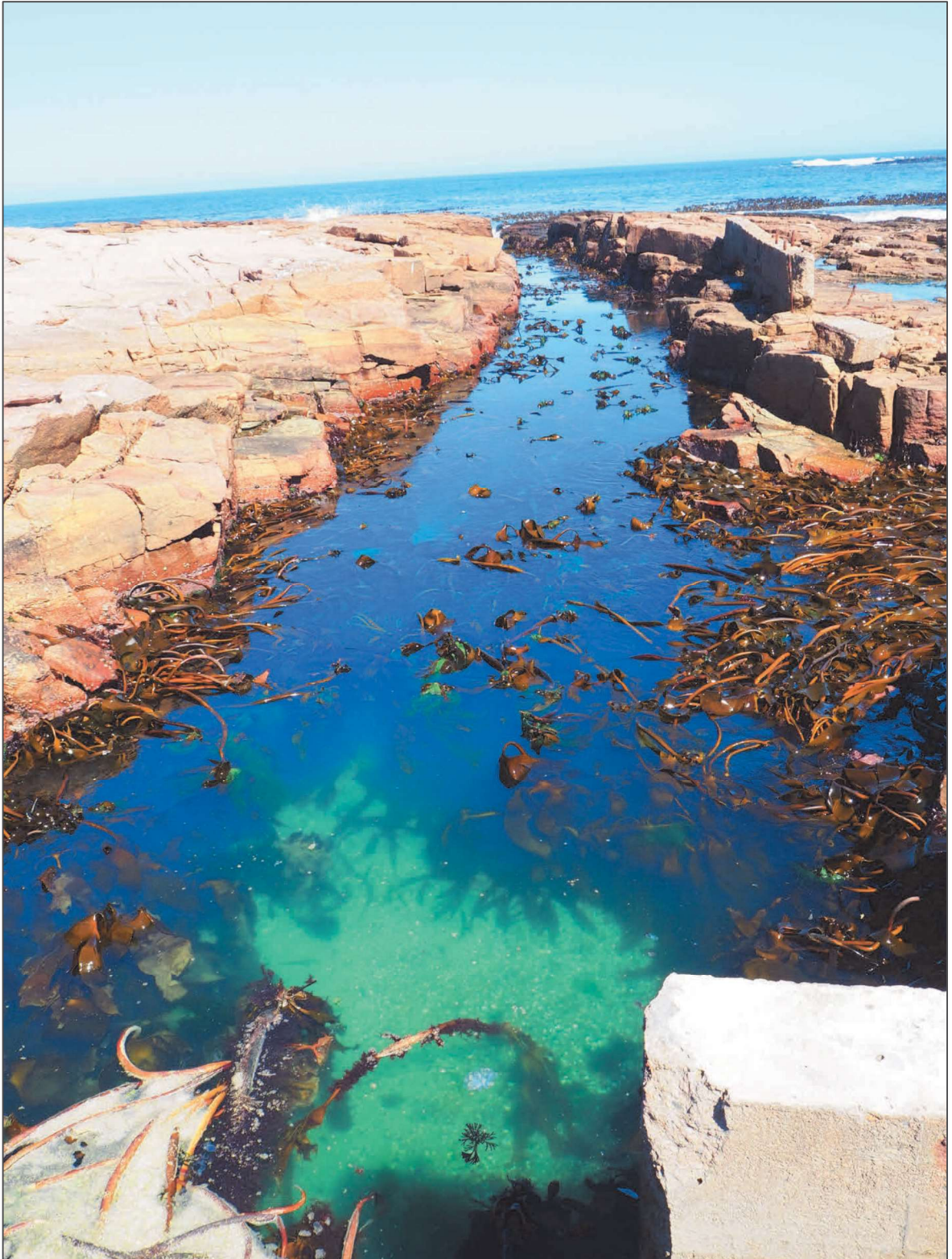
Figure 12. Feeder canal blasted through coastal rock
