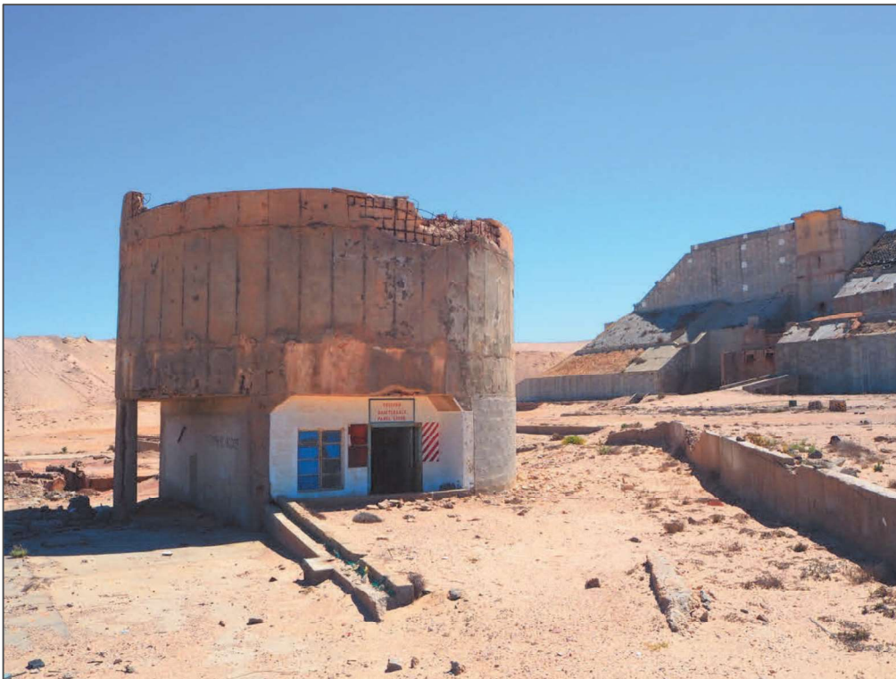
Figure 21. Maintenance Panel Store
