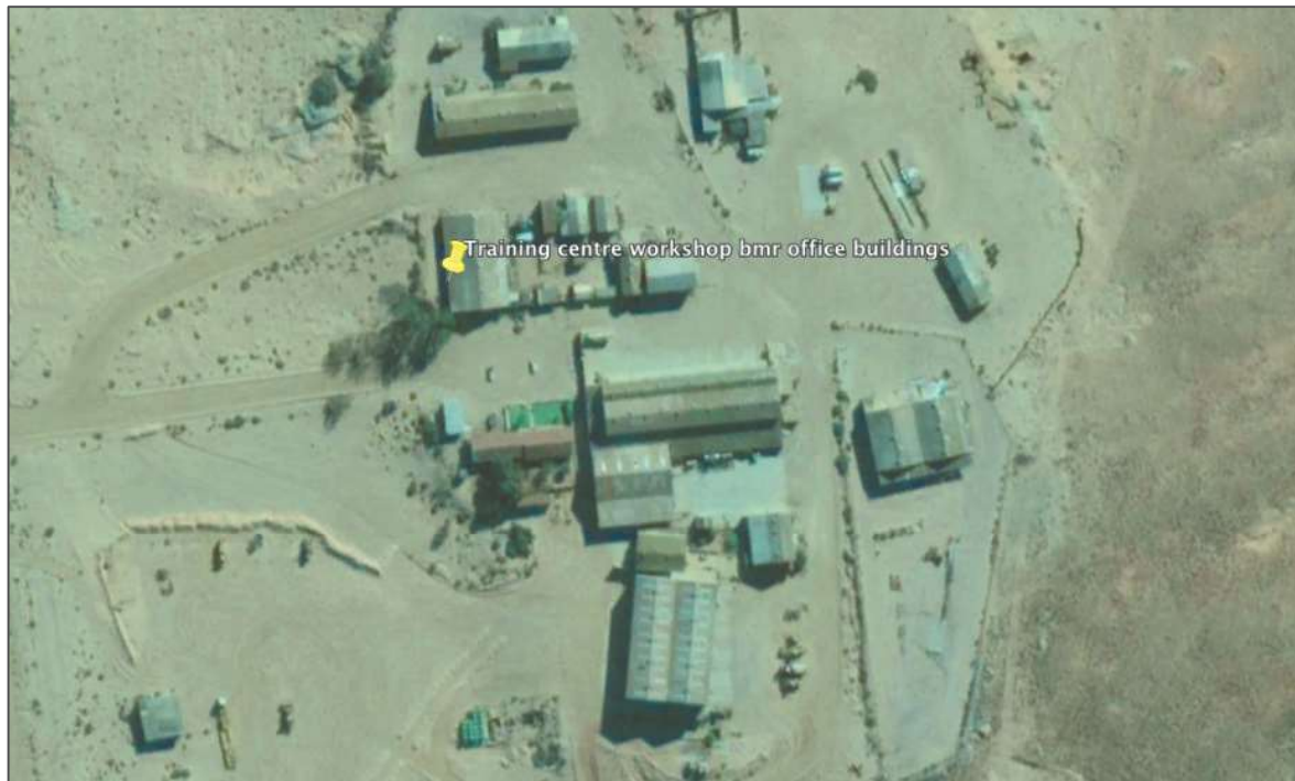
Figure 34. BMR Workshops and Mine Offices
