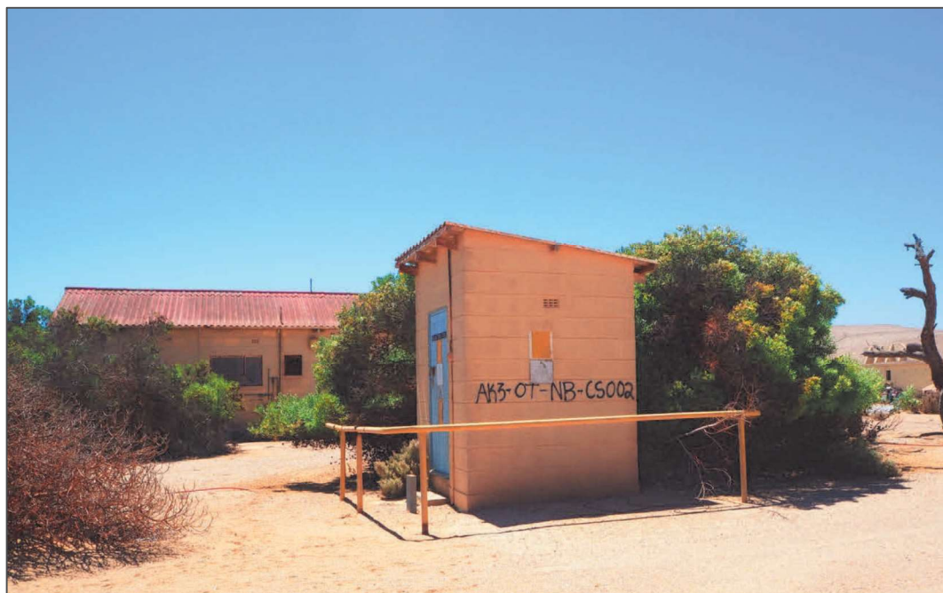
Figure 51. AK3 Office Block and Sub Station
