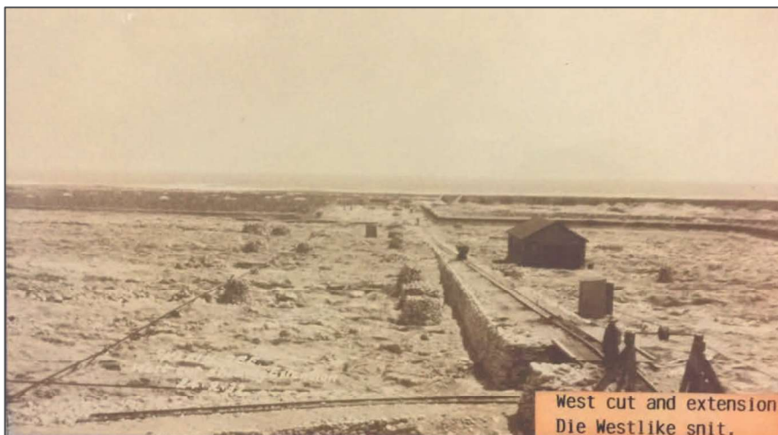
Figure 6. Western Mining Cut
