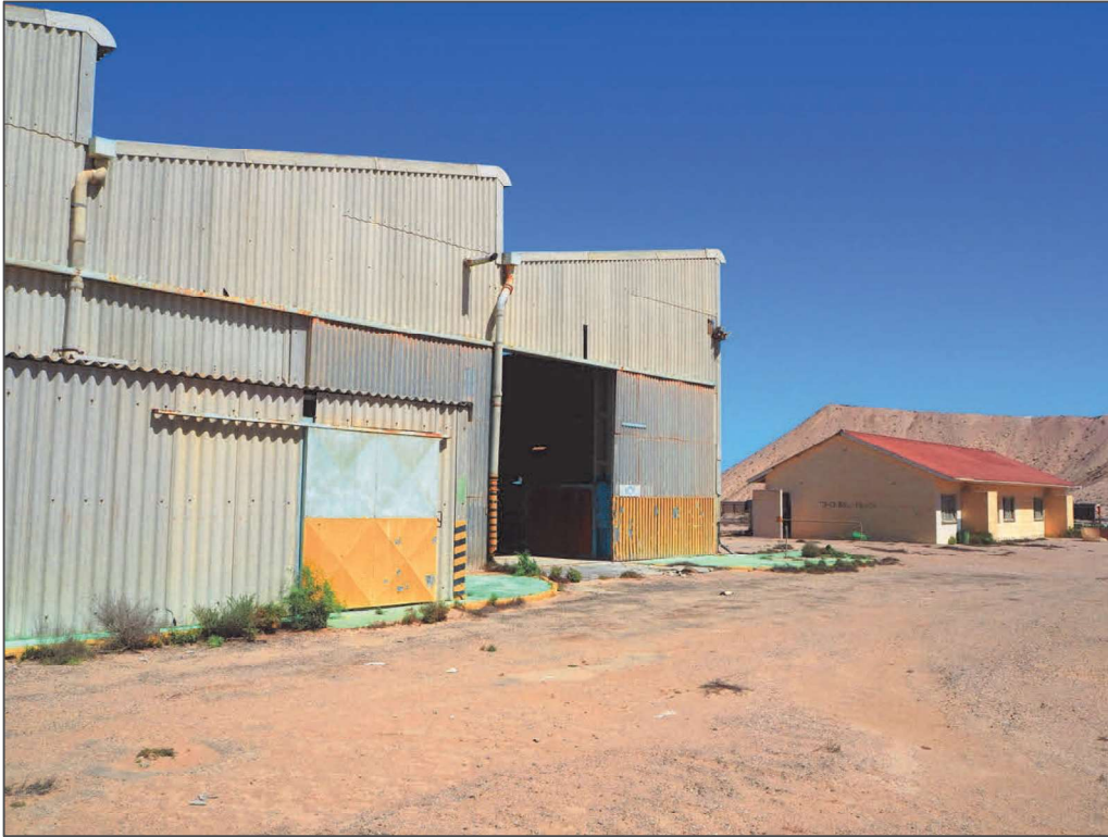
Figure 16. Steel and Asbestos shed and offices
