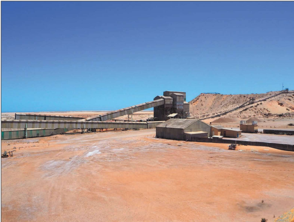
Figure 29. Bulk Sampling Plant with Conveyor System
