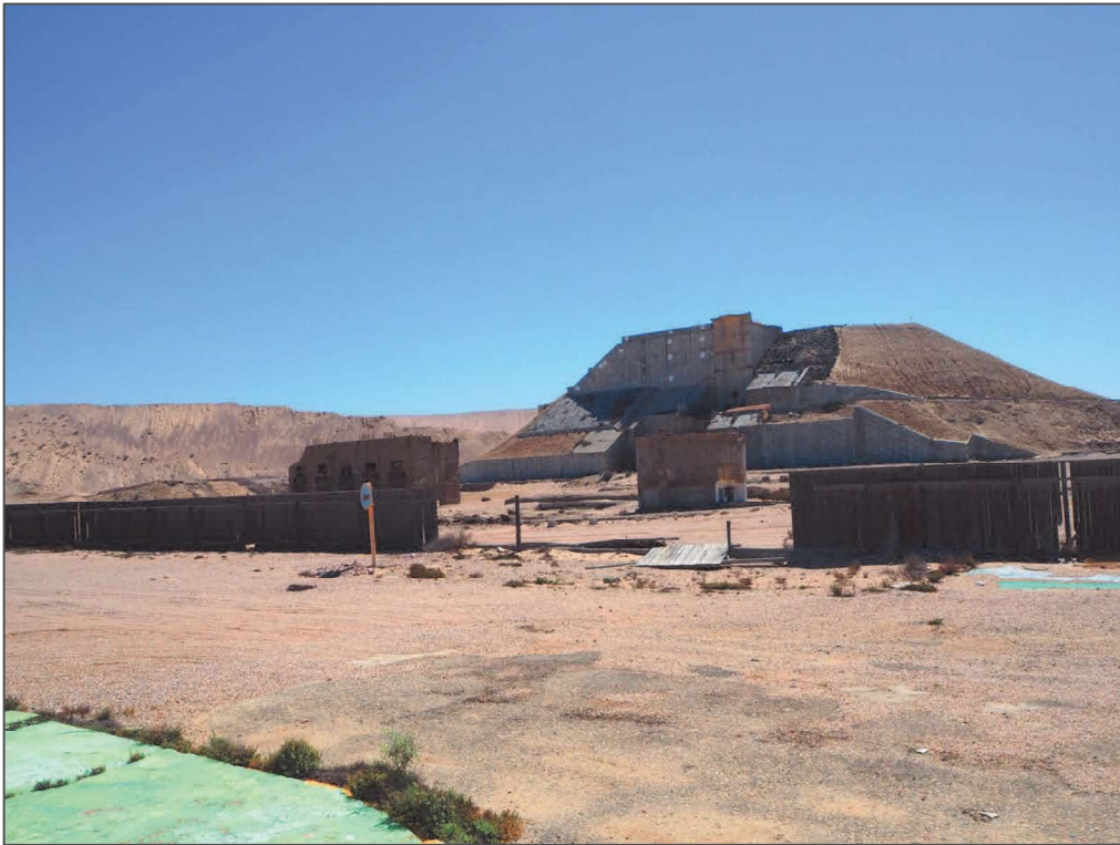
Figure 18. Dump site with retaining wall
