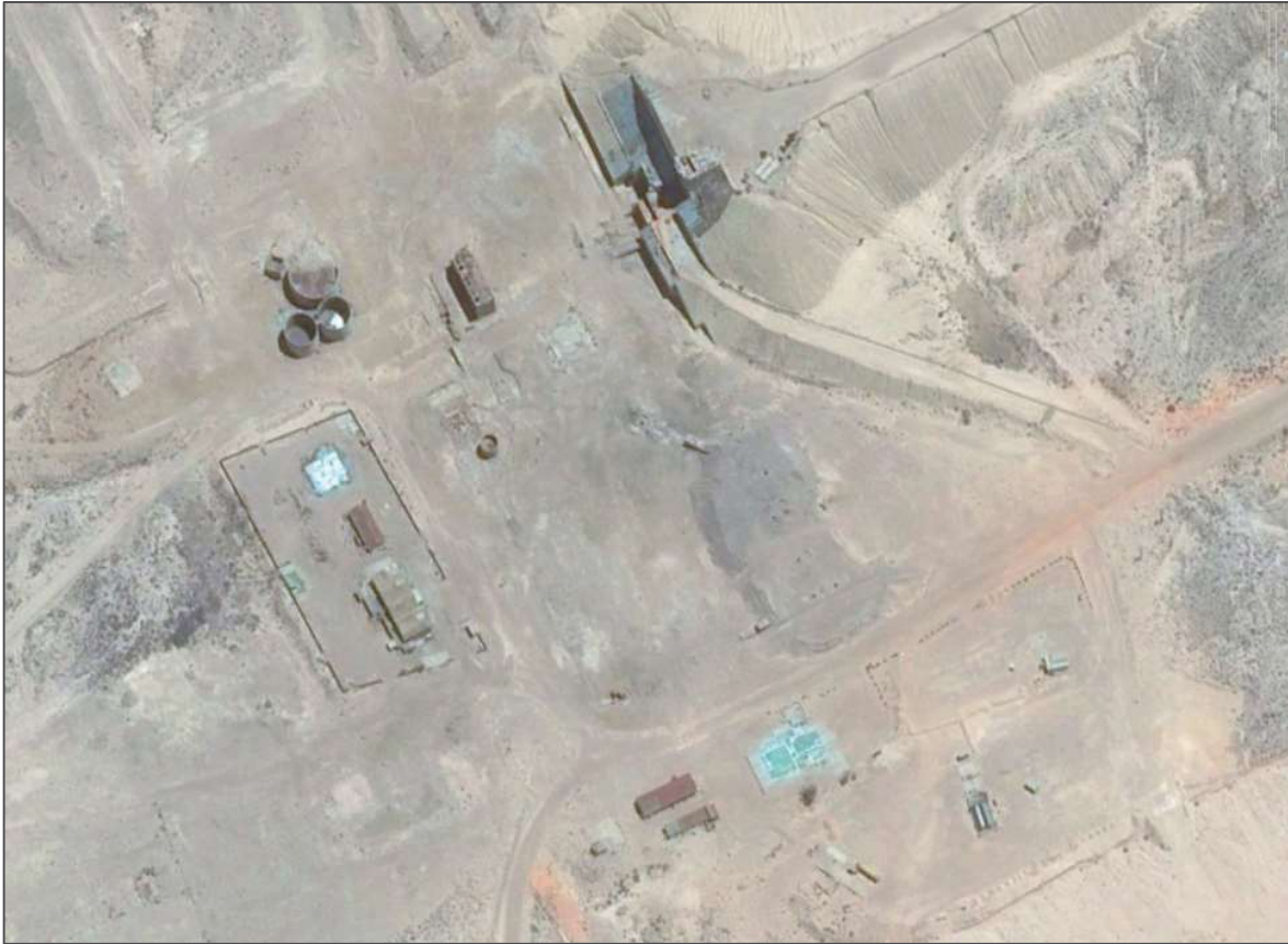
Figure 15. Tweepad Processing Plant
