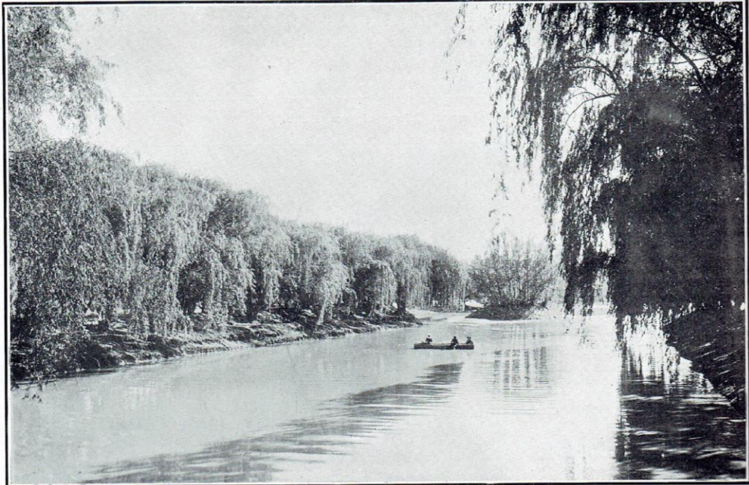
Figure 13: General view of the lake in 1905
