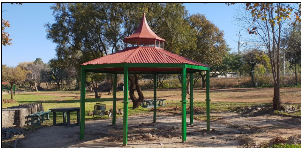
Figure 8: General view of an existing pagoda being restored
