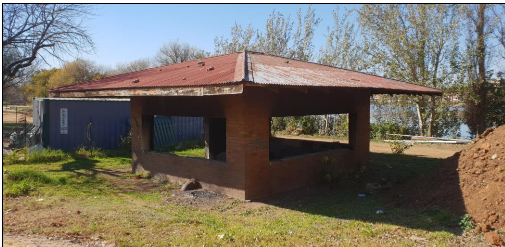
Figure 11: Existing square brick structure with corrugated iron roof
