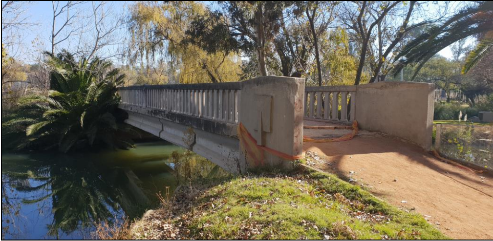
Figure 6: General view of the eastern section with a bridge
