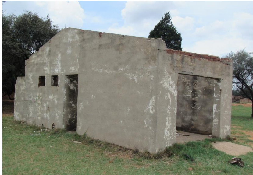
Figure 35 –The remains of the recent house
