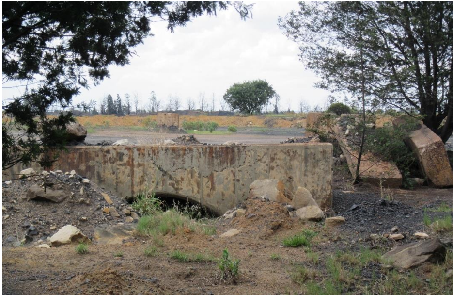
Figure 29 – View showing some of demolished remains
