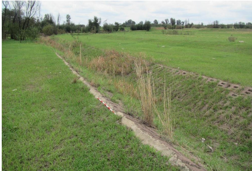
Figure 27 – View of the ditch
