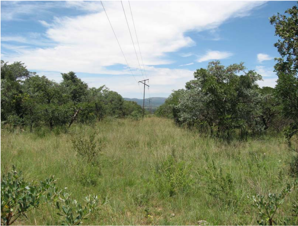
Photo 3: View of the power line across the site.
