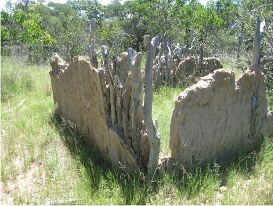
Photo 9: View of the mud and pole construction technique at site 24R 003.
