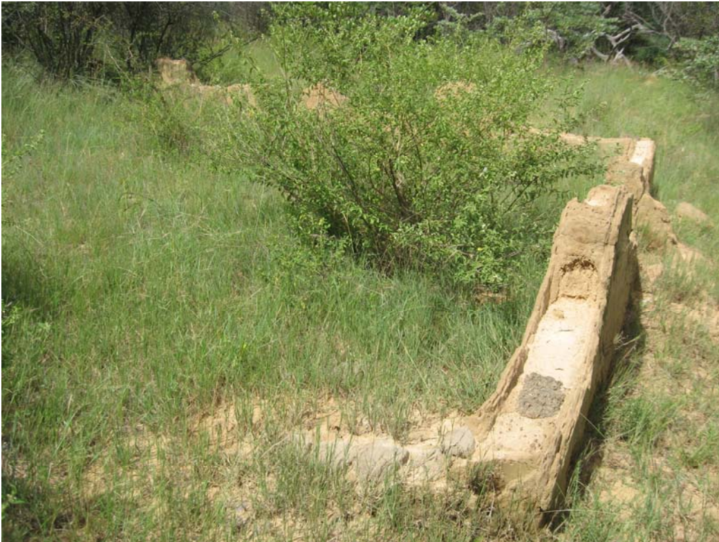
Photo 14: View of the mud brick walls at site 24R 005.
