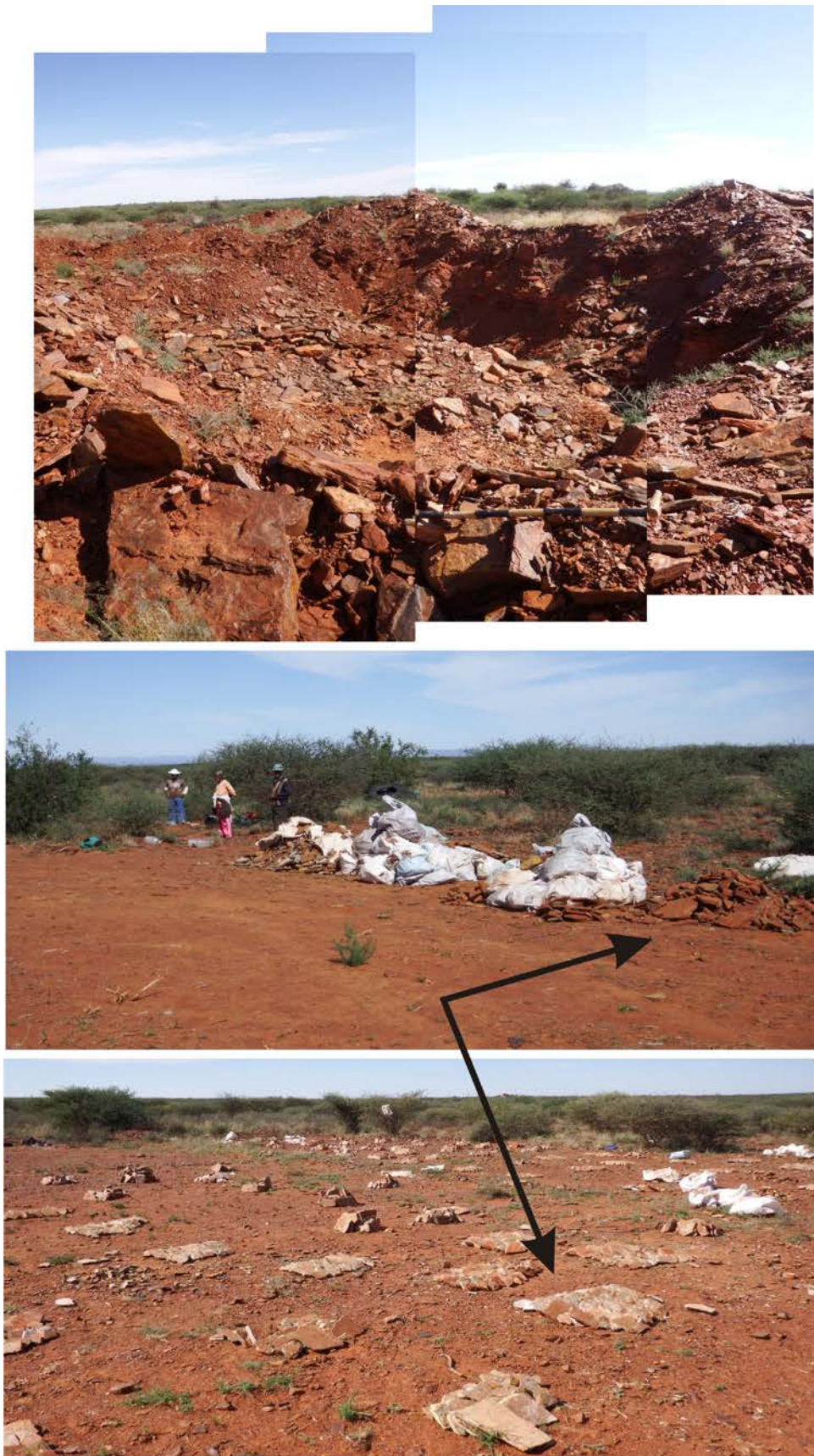
Figure 7. Existing mining activities (top) and excavated material (center and bottom).
