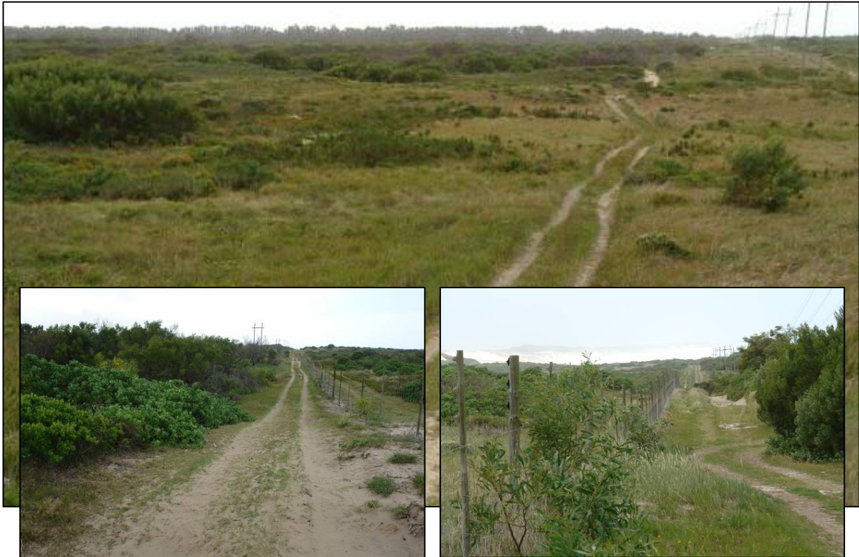
Figure 5. General views of the sludge pumping main route where it follows the boundary fence of the Nelson Mandela Metropolitan University's property in a northerly direction.
