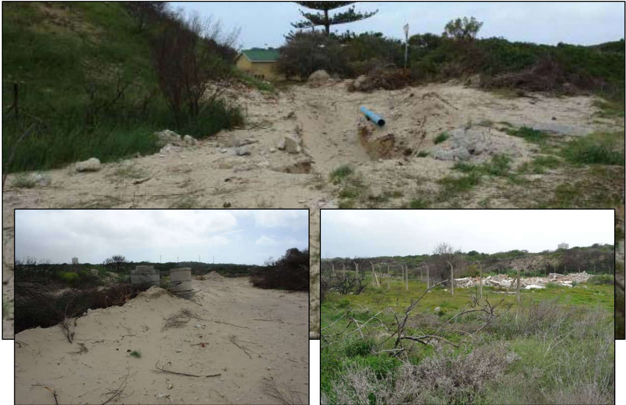
Figure 1. General views of the sludge pumping main route from the Cape Recife WWTW to Marine Drive. Note the disturbed nature of the area.
