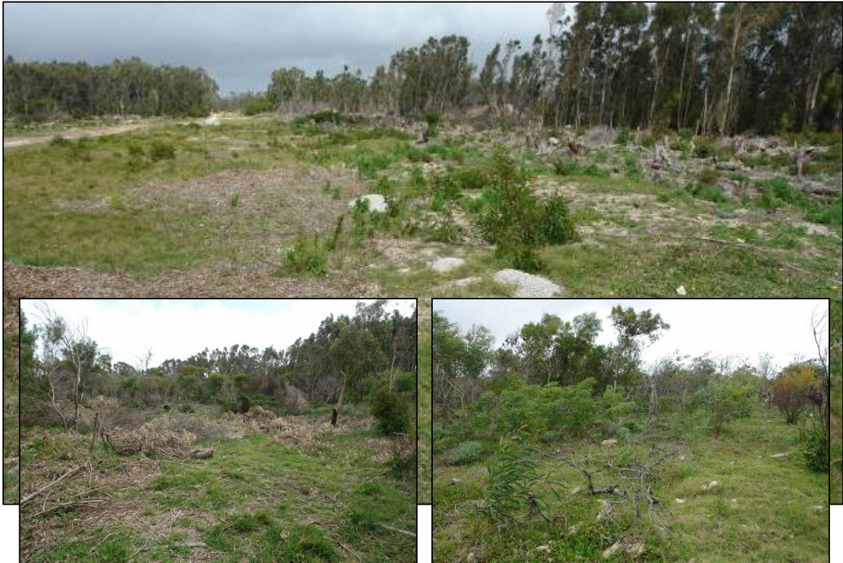
Figure 7. General views of the sludge pumping main route where it follows an existing pipeline route and track in a south-westerly direction towards the the Driftsands WWTW. Note the dense alien vegetation.
