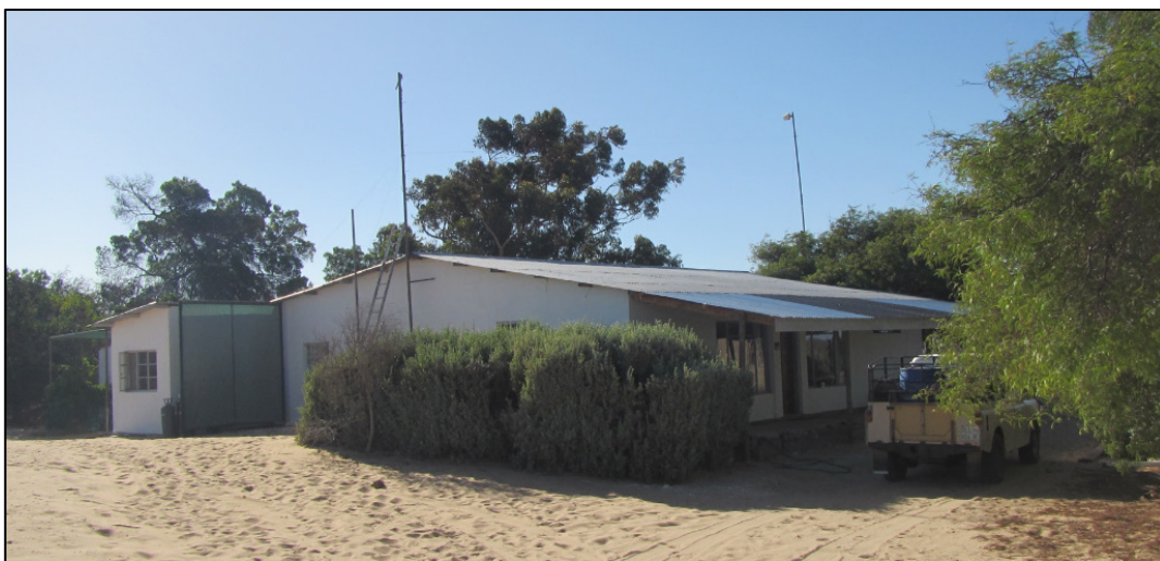
Figure 24: Farm house on Farm 128/4 to the west of the site (photographed in 2018).
