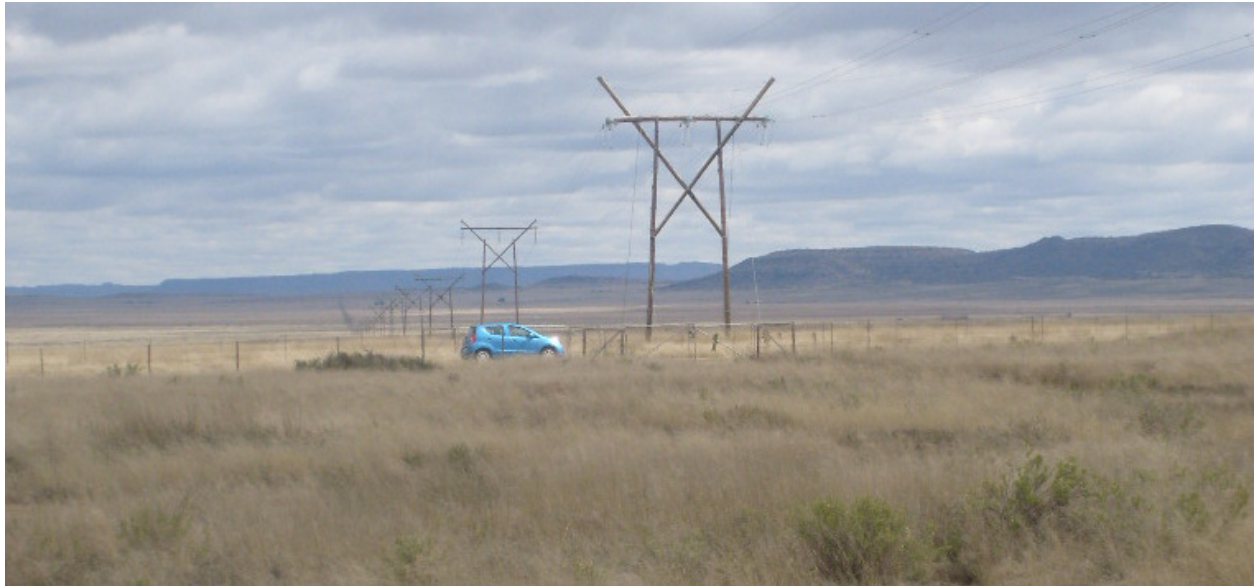
Photograph 1: Vegetation and Existing Power Line
