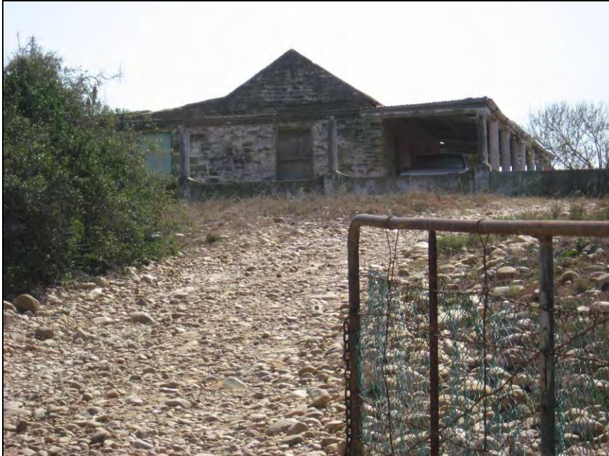
Fig. 24 -25 Early farmhouse circa 1890 S33 44 056; E25 35 249 with stone gables and an added verandah (probably 1920's) (Photos: J S Bennie)
