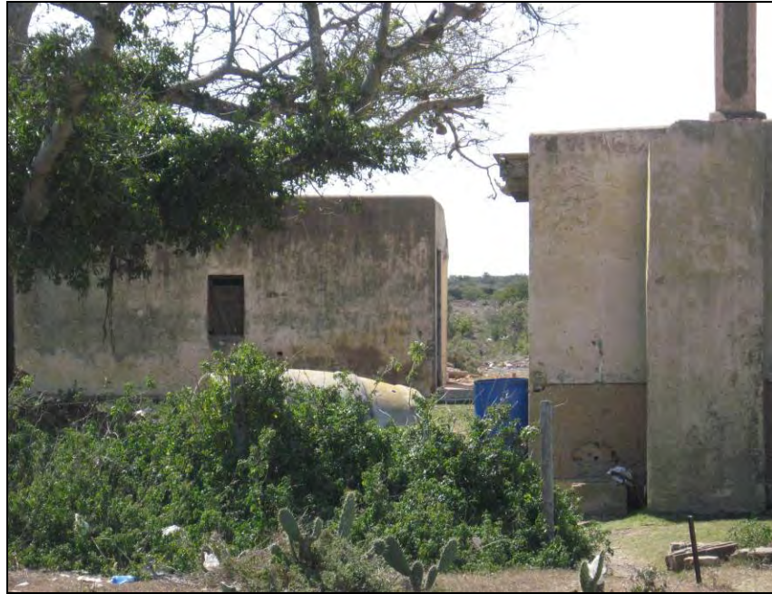
Fig 22 Water tanks, tree and outbuilding (Photos: J S Bennie)
