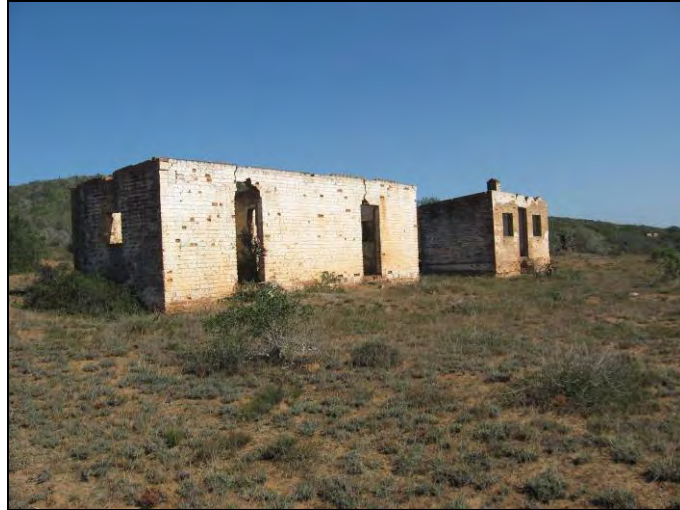
Fig. 6 Two derelict labourers' cottages (Photo: J S Bennie)
