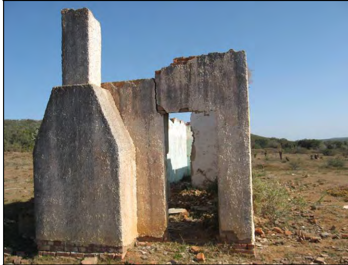
Fig.3 Chimney flue and back door (Photo: J S Bennie)
