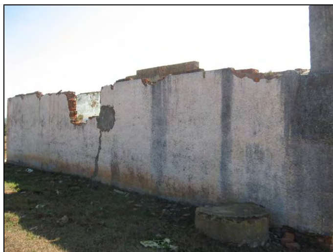
Fig.5 Back wall and water tank (Photo: J S Bennie)
