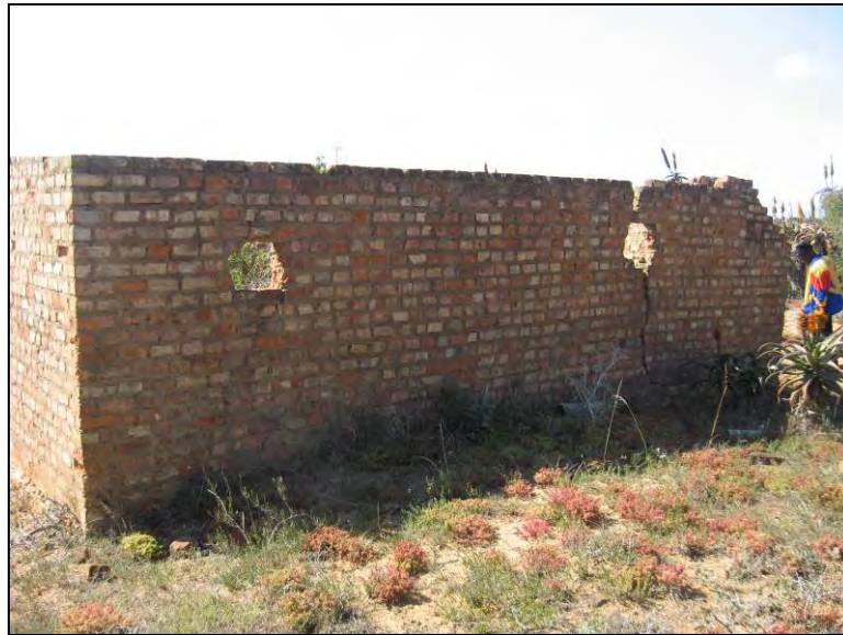
Fig. 14 Rear view of labourer's cottage showing two small windows
