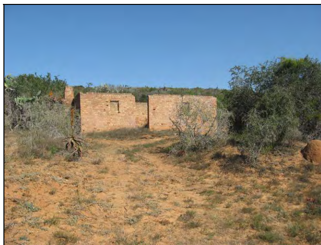
Fig.18 West view of cottages (Photo: J S Bennie)
