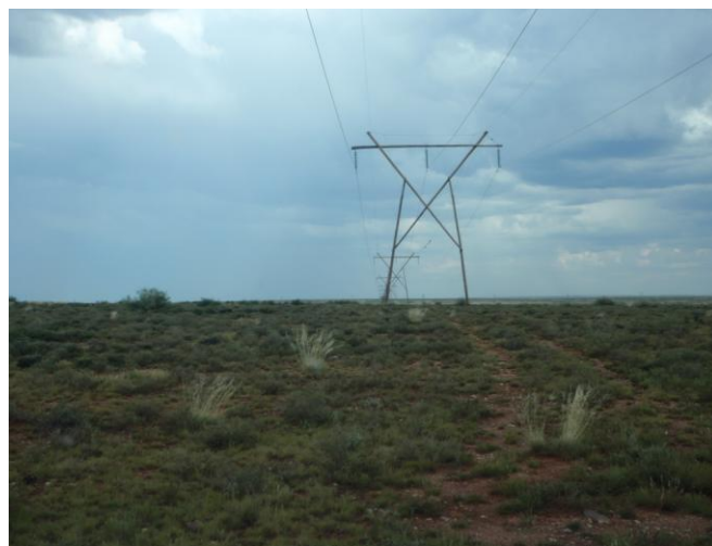
The site looking north east showing the existing overhead pylons
