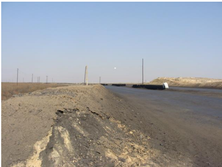
Figure 6: Mine road along which a short section of the proposed North Road will run.
