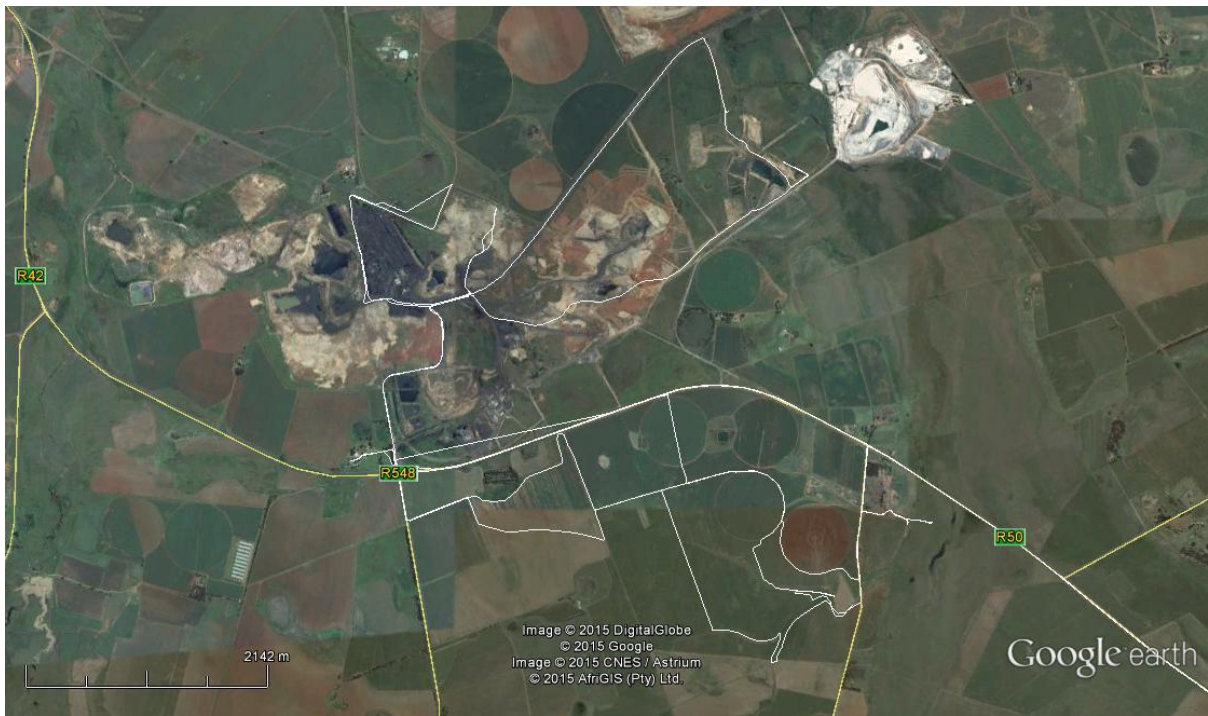
Figure 4: GPS track route of the R50 survey 4 . North reference is to the top.
