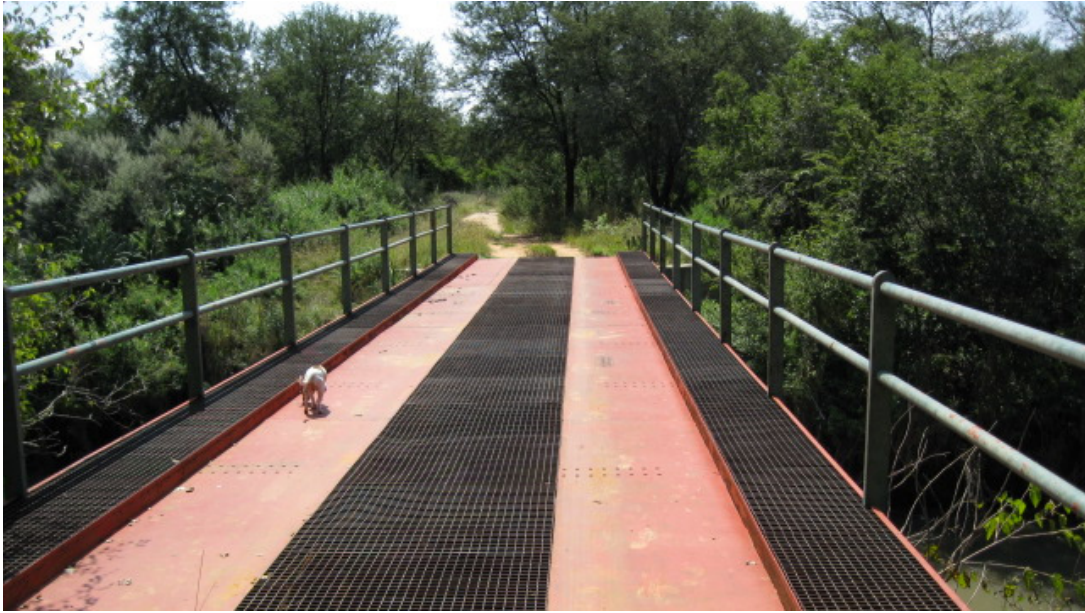
Bridge to the Property under investigation.
