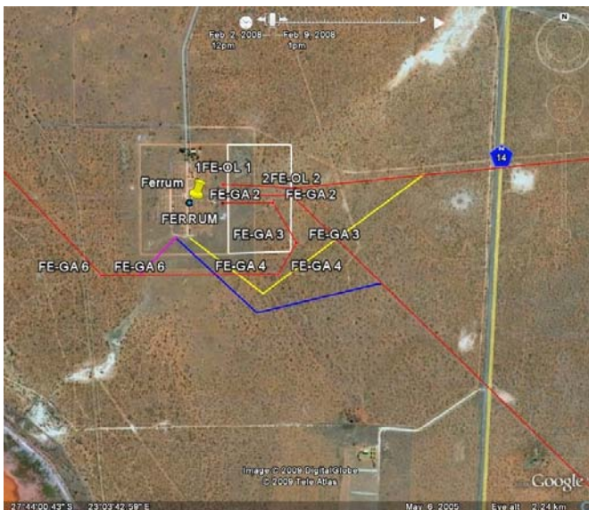
Fig. 1 Ferrum Substation (Map provided by client). The area that was assessed is approximately 1 km around the existing substation.
