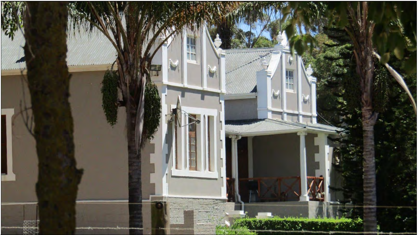
Figure 12: The homestead at Farm Werf 1 on Rem Farm 830 graded IIIB
