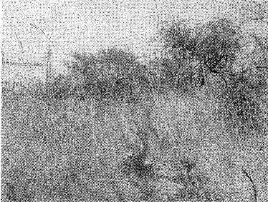
Figure 4 The Legogote Switching Station where both routes end. Note the dense, but disturbed vegetation.
