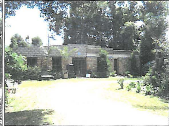
Building used as antique and woodwork store
