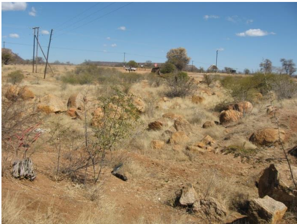
Figure 6 – View of the dumped rocks in the small stream.
