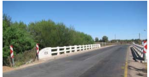
Plate 3. Bridge 2464 (looking south)
