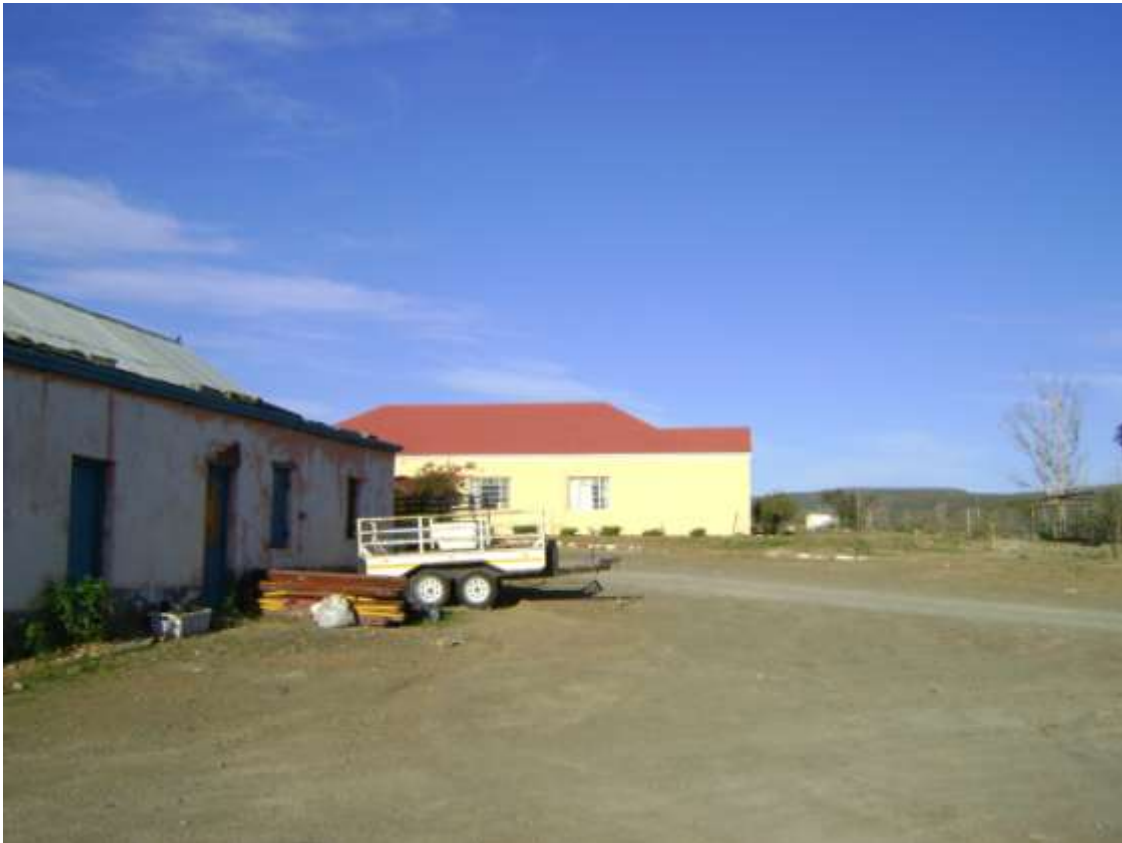
• Photo 8 Old Barn
