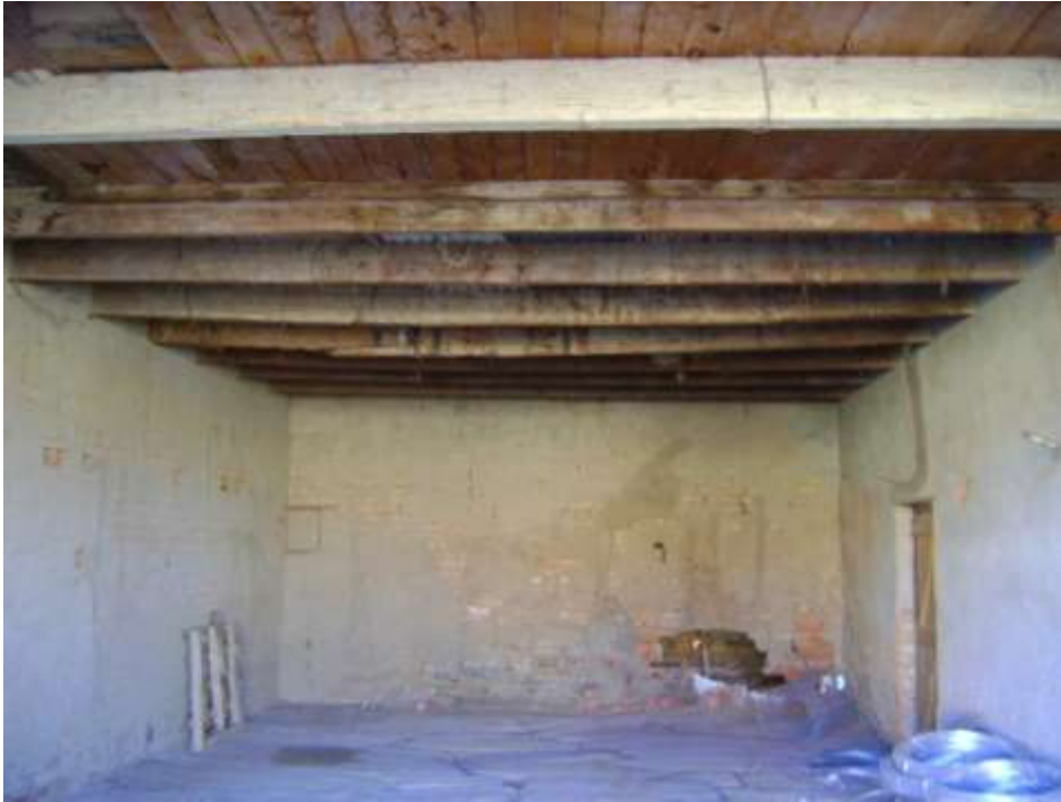
• Photo 11 Interior of structure
