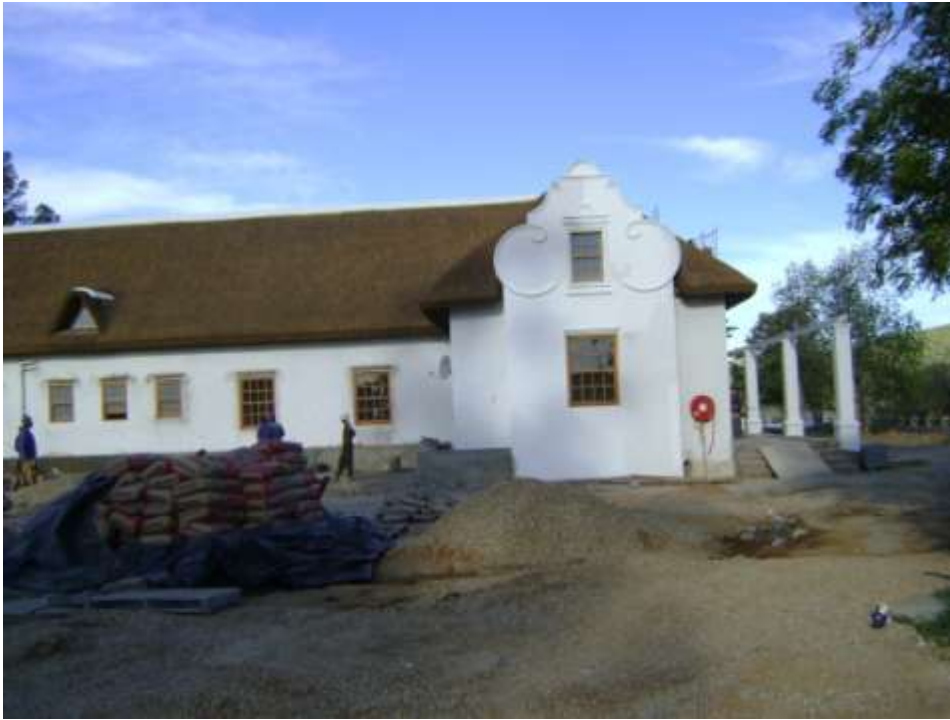
• Photo 1 Renovated Farm Homestead
