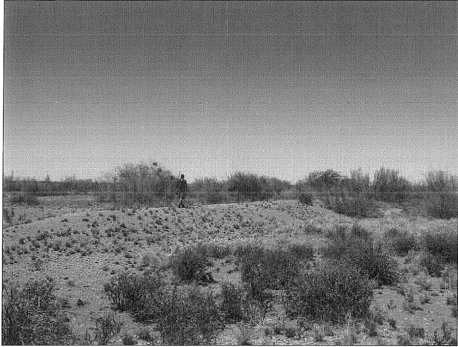
FIGURE 9: Earth retaining wall constructed across the dry river bed at Site 5
