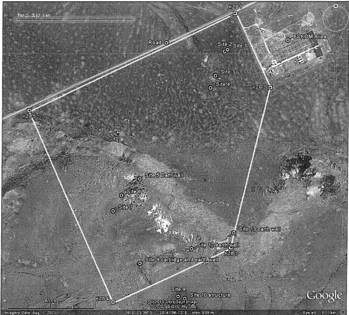
FIGURE 7: Google Earth image (2005) of the development area indicating the archaeological and historical sites that were investigated in some detail
