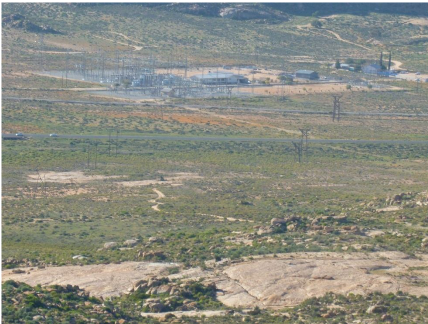
Figure 7: The power line corridor looking towards the substation
