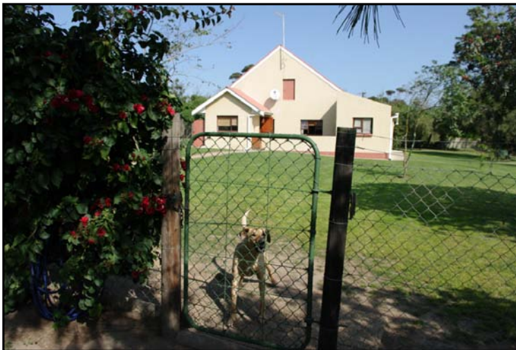
Figure 19: View of the Site 1.4 Zeekoe River farmhouse
