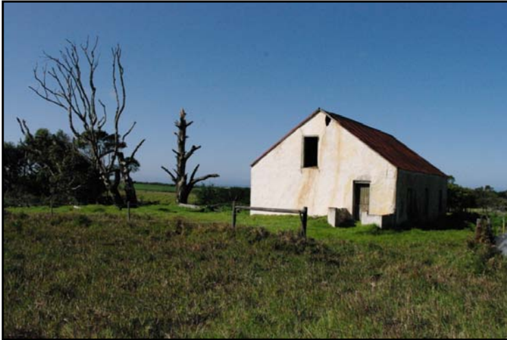
Figure 40: View of the Site 2.4 Welgelegen farmhouse, also recorded by Anderson (2010) as Site MEL 07 and photographically documented by the ACO UCT (2010:47)
