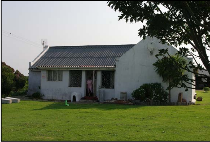
Figure 30: View of the Site 2.1 Colonial Period Welgelegen farmstead
