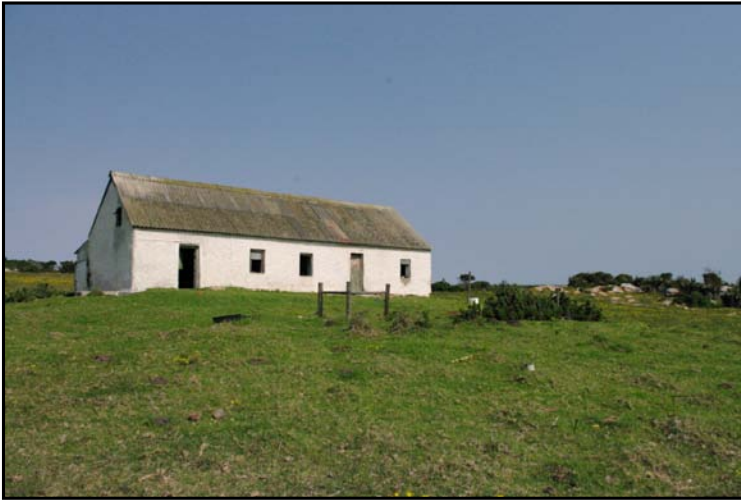
Figure 42: View of the Site 2.6 main residence
