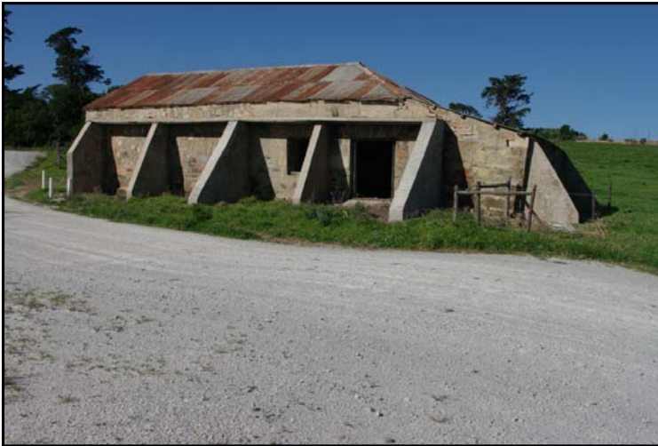
Figure 55: Site 3.1 - Colonial Period storage facilities; formal conservation of the structure is not recommended based on proximity to the road and landowner usage requirements
