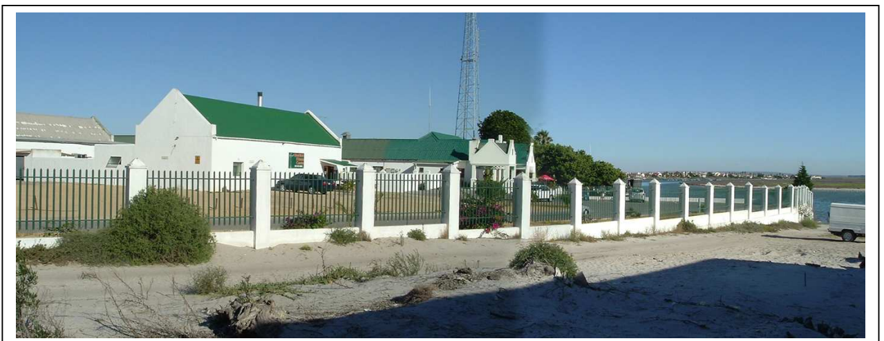
Historic Core – West facade from Erf 478 passage to Berg River
