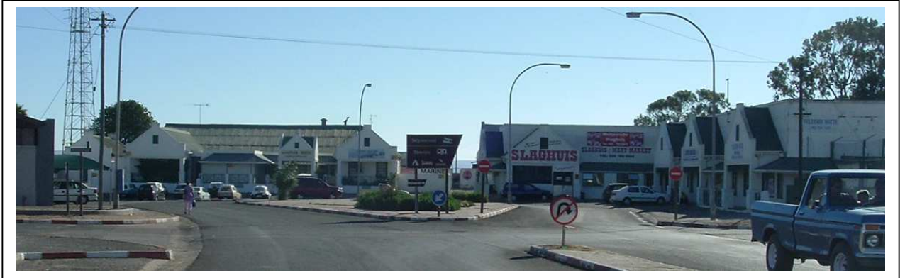
Historic Core – Laaiplek Hotel (Left), village square foreground, old Anglican church behind the butchery (centre right).
