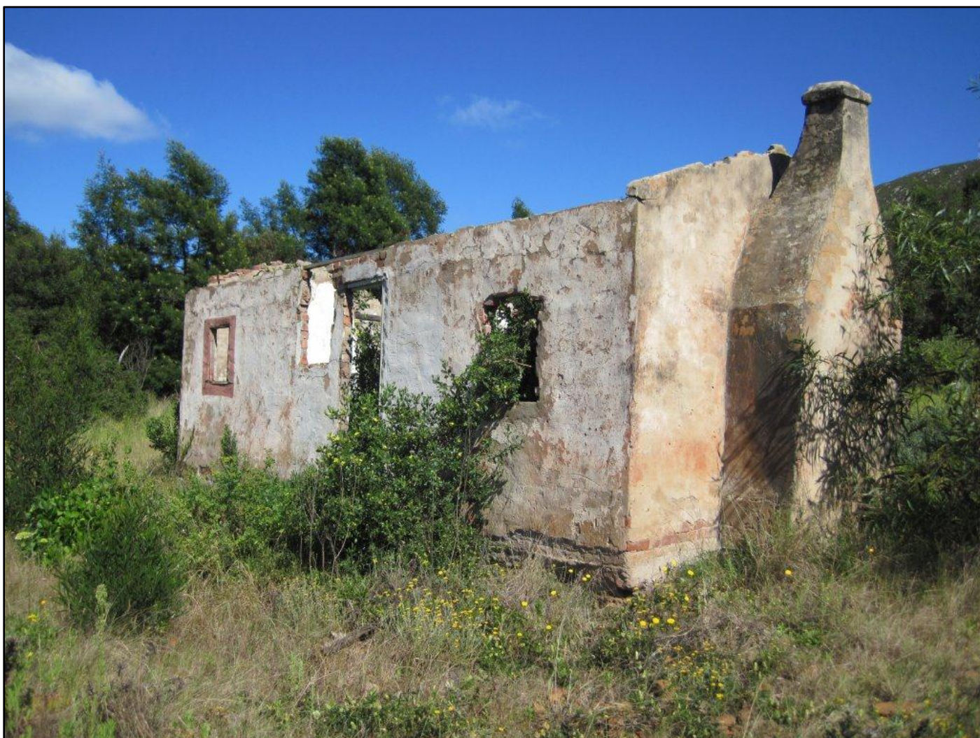
Figure 7 – View of structure on site
