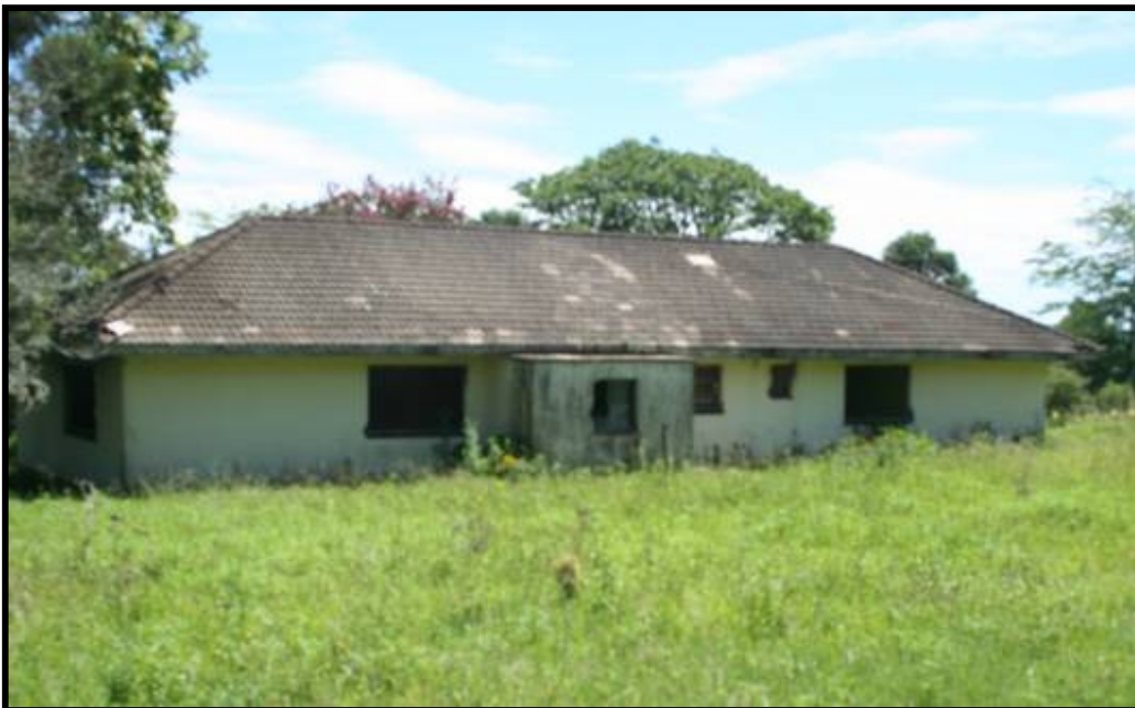
FIG. 10 ABANDONED HOUSE AT BER03.1
