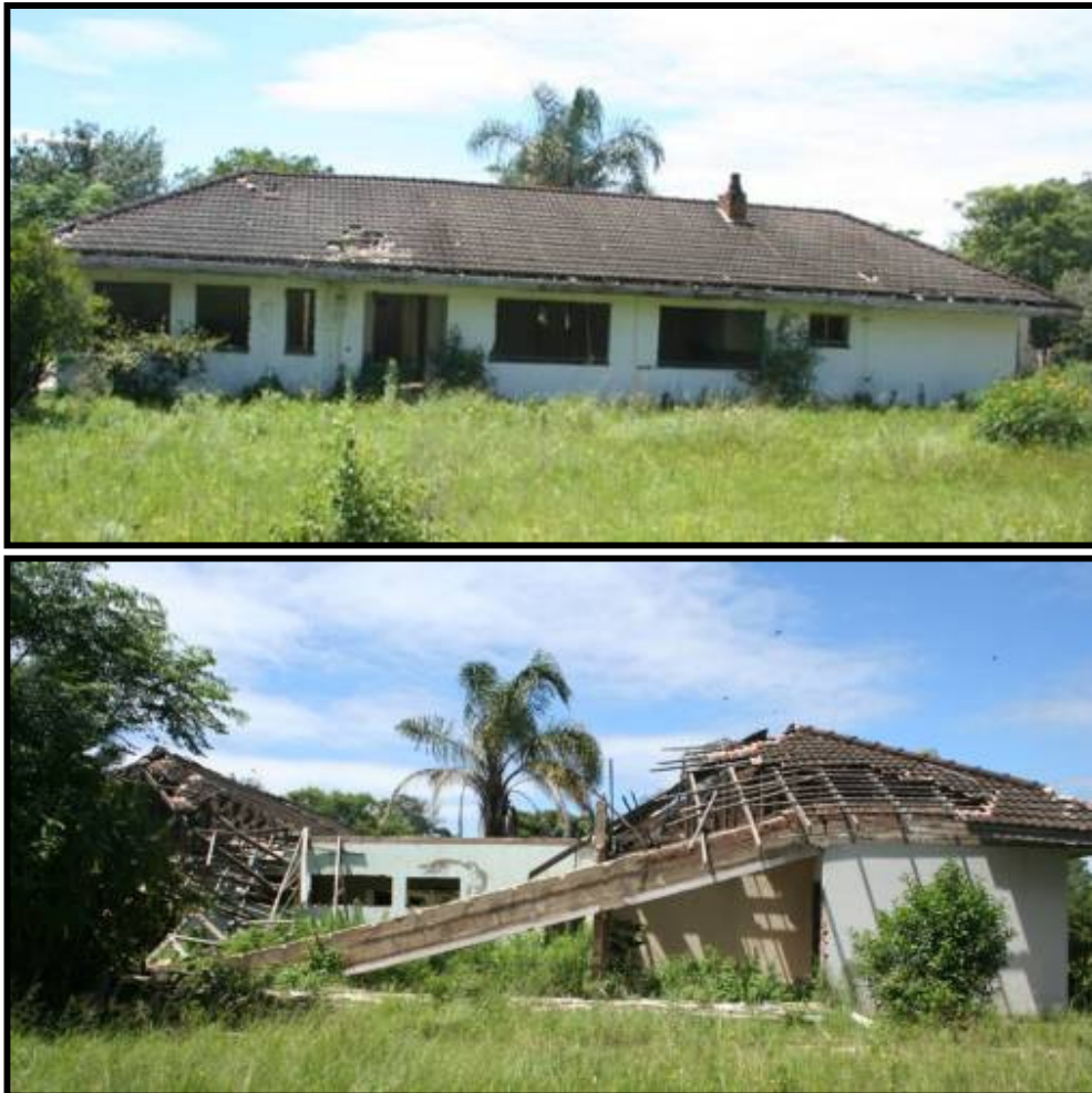
FIG. 9: ABANDONED HOUSE AT BER03
