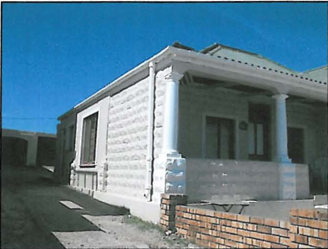
Figure A2: Side view of the house at 116 Beach Road.
