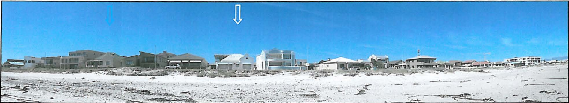
Figure A3: Panoramic view of the beachfront with 110 Beach Road indicated by the white arrow. The similar house at 116 is indicated by the blue arrow.
