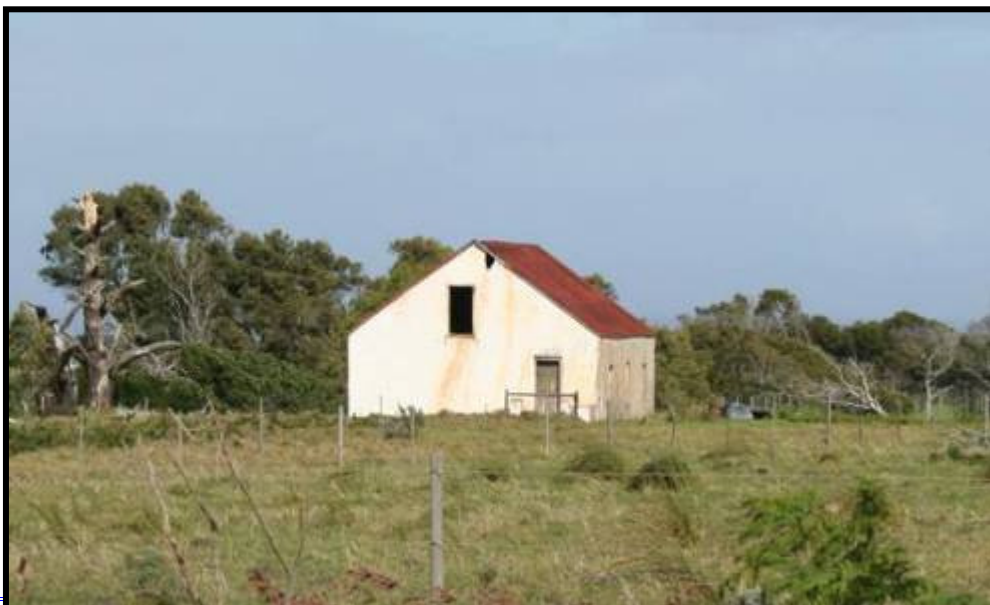
FIG. 8: OLD FARM BUILDING
