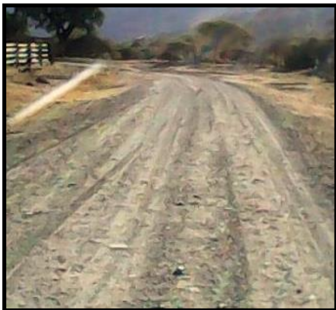
Figure 6. Photograph of the existing track at Mlindazwe Road, Msinga. No heritage features occur in the near vicinity of this track.
