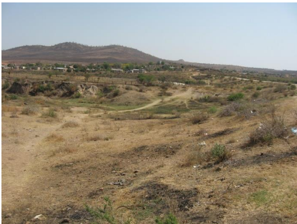
Figure 17 - View of the Dithokeng Dam Wall proposed Pipeline Crossing.
