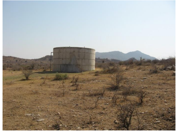
Figure 13– View of the existing reservoir and the location of Tshamahansi Reservoir C.
