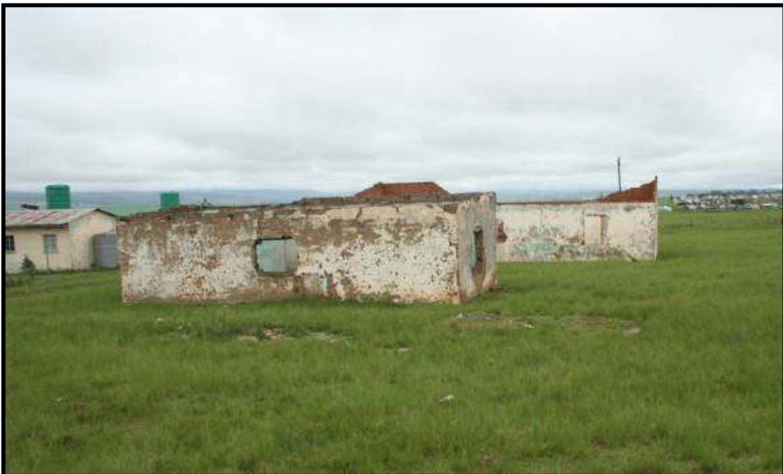
FIGURE 7: ABANDONED BUILDINGS AT NCO2
